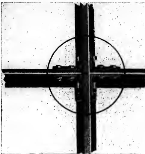
The gable posts are flat bar steel like the roof rafters. The gable purlins are steel angles. The purlins are bolted to the posts by double angle plates. DOUBLE , mind you. Not single. TWO bolts are used on the purlins. Two , mind you. Not one. Each gable bar is screwed to each purlin.
