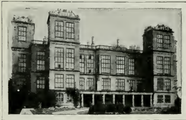
Abb. 148. Hardwicke Hall, Derbyshire.
