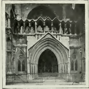
Abb. 212. Law Courts, Portal am Strand. (Street.)
