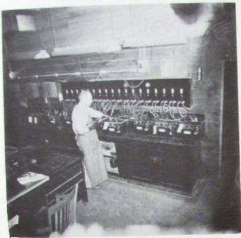
BATTERIES NEED CHARGING
