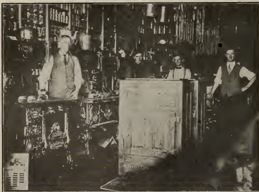
Part of Griffin & Brennan's Store, Arnprior—Had the Counter Not Been Removed There Would Have Been No Room for the Stoves.
