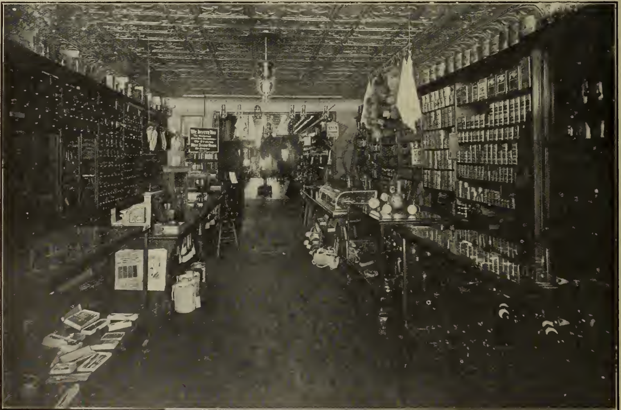
A view of the main floor of the store of Geo. A. Elliott Jr.—The gas stoves are kept in the rear section—a good selection is always shown.
