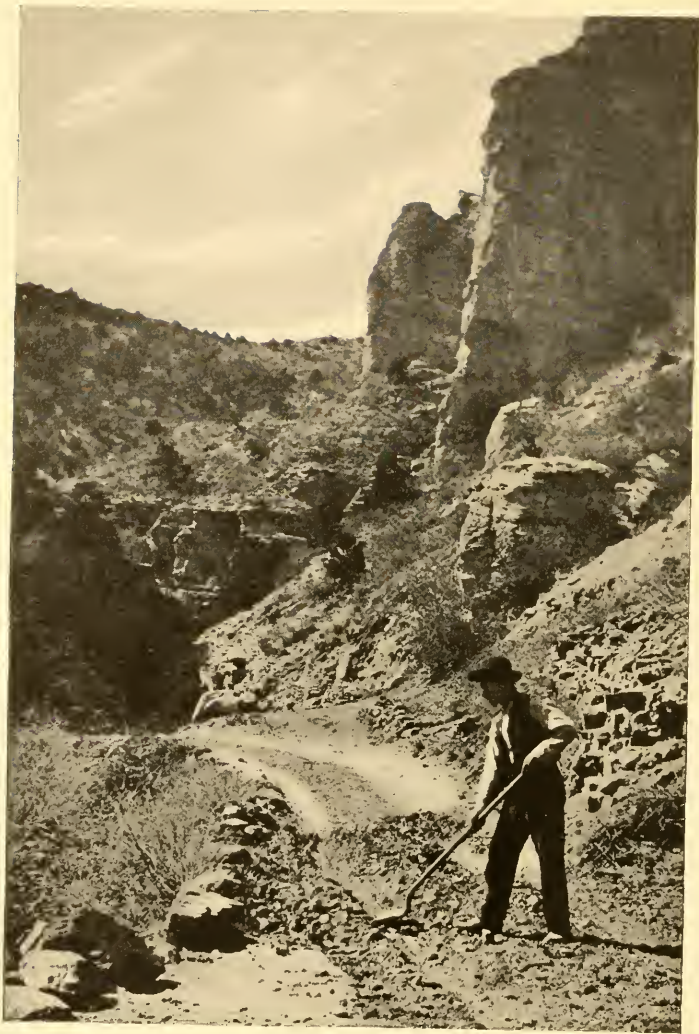
Working on the road
