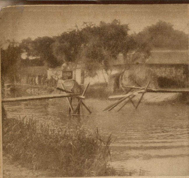
橋樑被炸燬後 When a bridge was destroyed.
