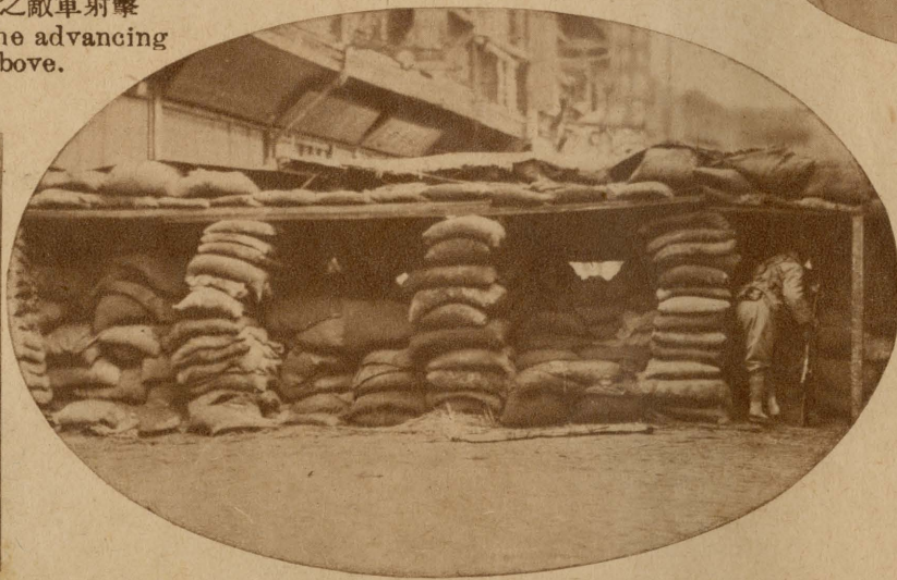
十九路軍之巷戰防禦工程 Defense work for Street Fight.
