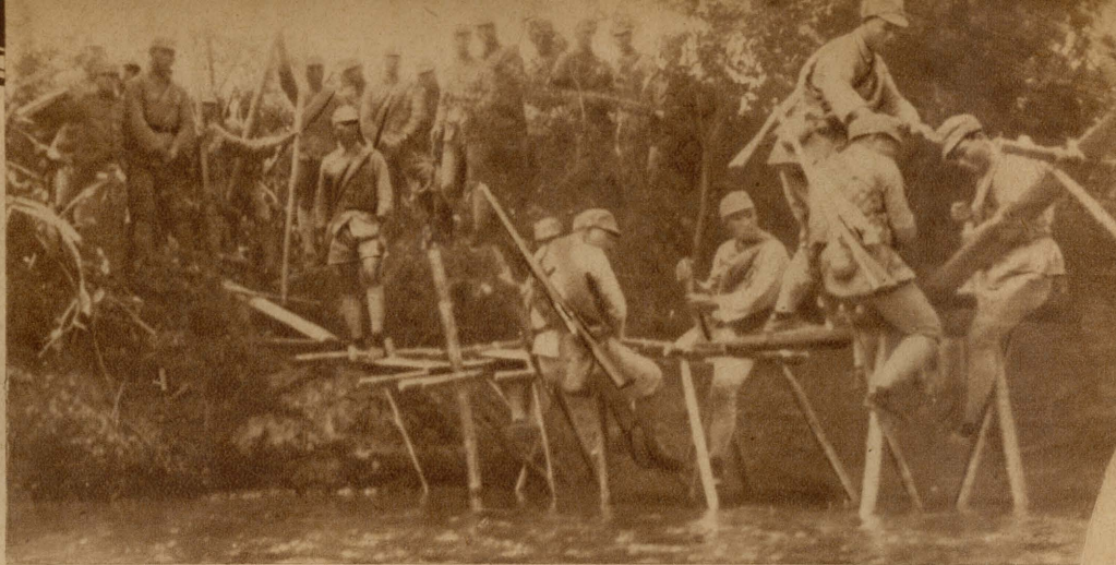
The pontoon-bridge set up by the 88th D. on a creek near Miaohang.
