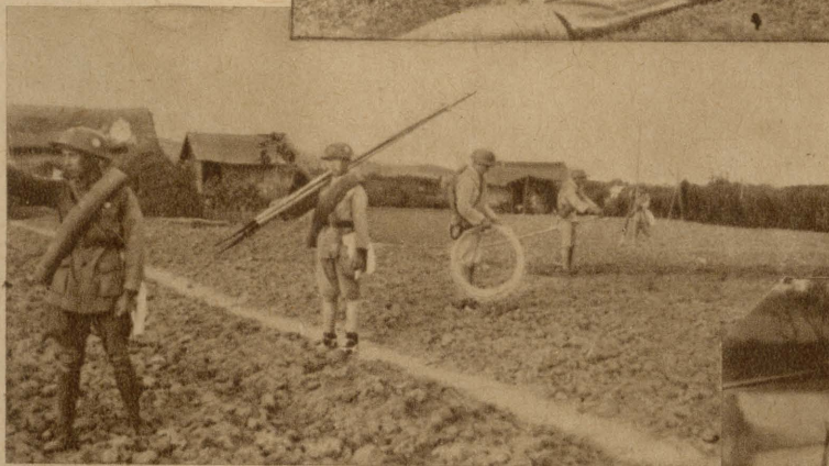
兩師通信營加緊作業一週內即完成全線之通信網 Engineering corps setting up telephone wire.
