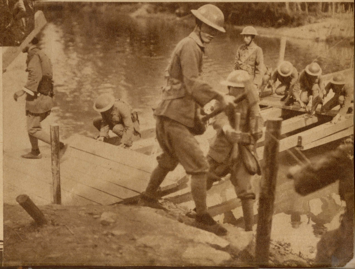
蘊藻浜上游浮橋之架設(八十七師工兵營) Setting up a pontoon-bridge on Wentsaopang Creek.
