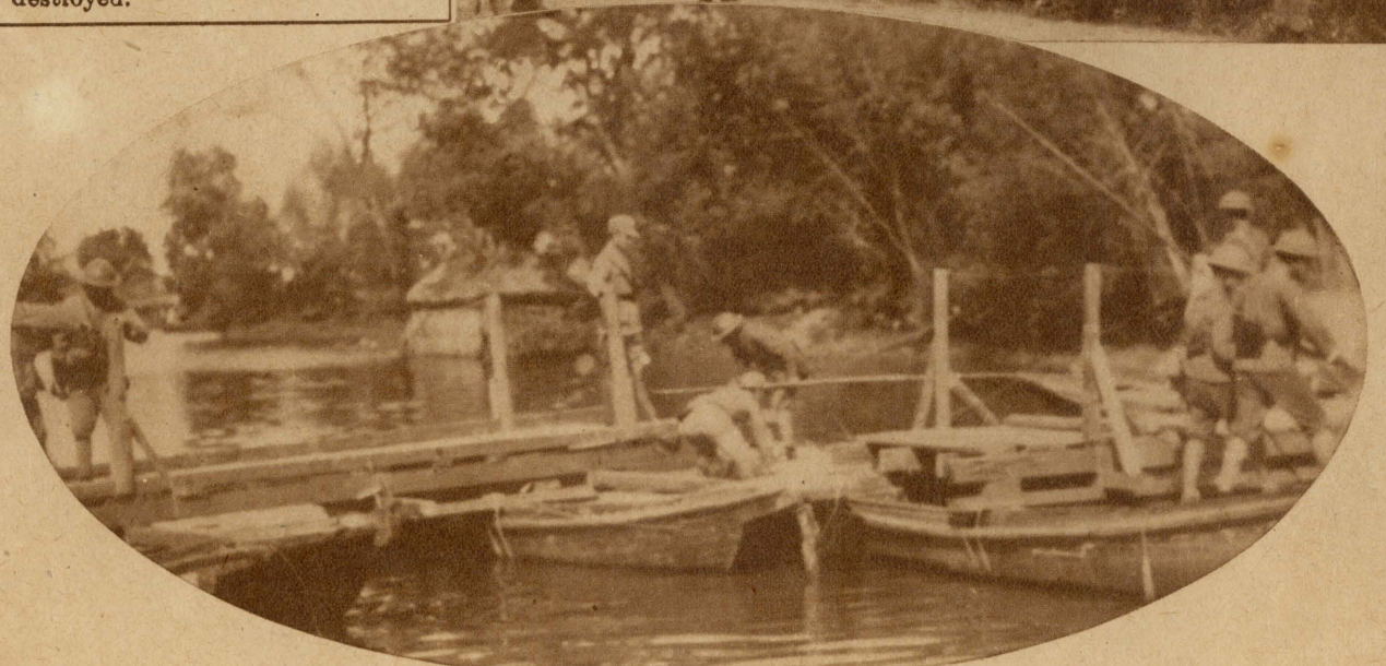
最後裝上橋門 When the pontoon-bridge was set up.
