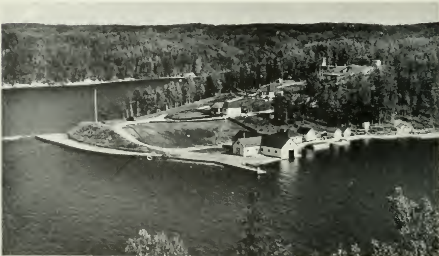
SKEAD RANGER HEADQUARTERS SUDBURY DISTRICT
