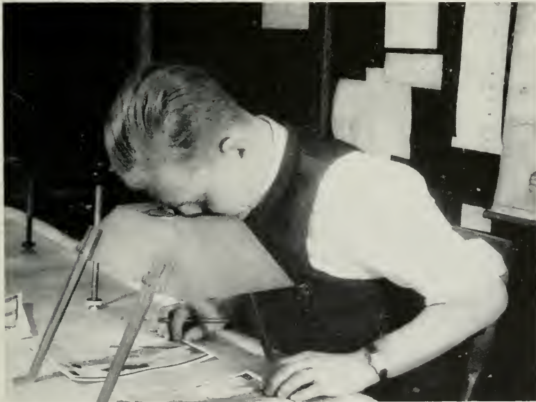
USING STEREOSCOPE In preparation of maps from aerial photographs.
