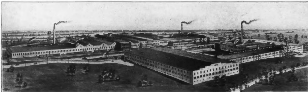
PLANT OF BOEHME & RAUSCH COMPANY, MONROE MILLS
