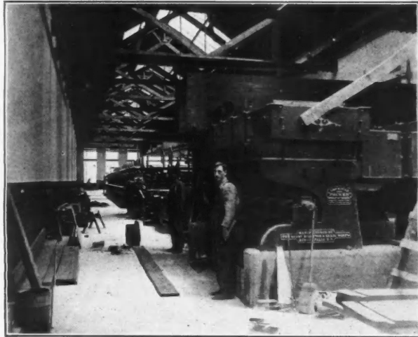
INTERIOR VIEW OF CERTAIN-TEED PRODUCTS CORP.
