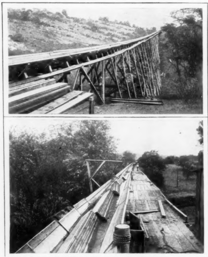
Two Views of a Sixty-Mile Flume, Built at a Cost of $3,000 a Mile, to Carry Lumber from a California Sawmill to the Railroad
