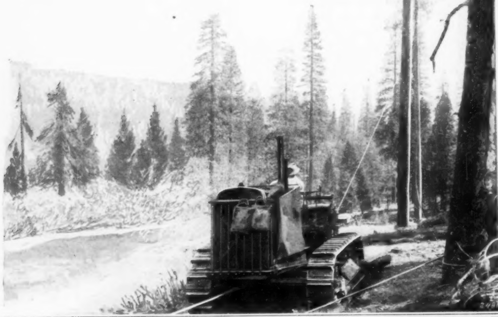
With the "Spar Tree" Set Up and Rigged, the Tractor Is Able to Handle All the Logs for 500 Feet Around, and Later Skyline Them to the Road or Railway
