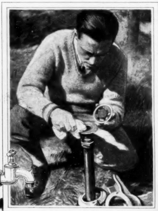
Left, Replacing Air-Dome Gasket; Center, Wiping Off Deck-Leather Seat; Right, Tightening Down Cylinder
