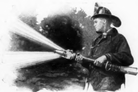
Nozzle Which Breaks the Force of the Fire Spray So That It Will Do Less Damage to Interiors
