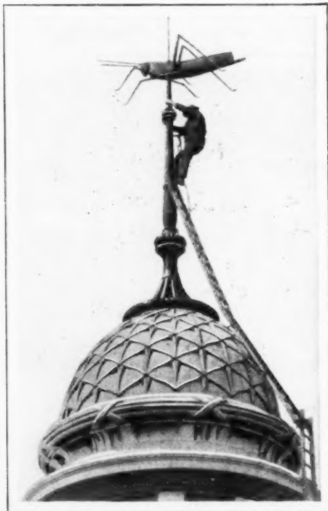
Cleaning One of London's Unique Weather Vanes; the Grasshopper on Top of the Royal Exchange
