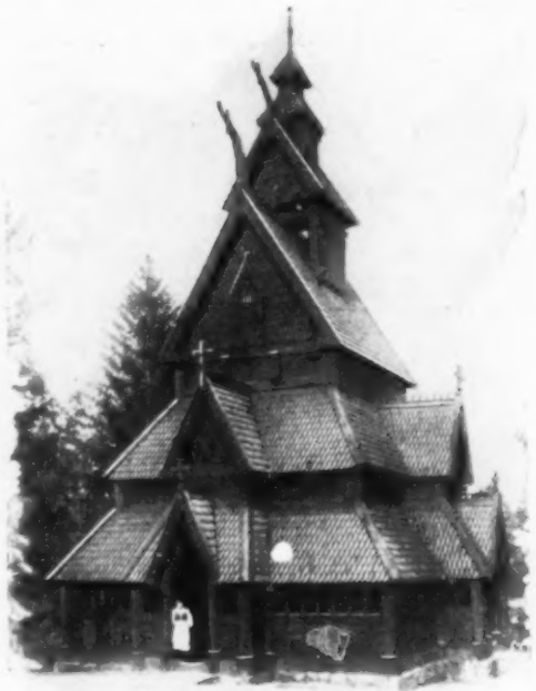
Glue and Wooden Pegs Hold This Norwegian Church Together; It Was Erected nearly 800 Years Ago
