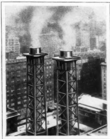
Steel Lattice around High Smokestacks, to Shield Their Unsightly Appearance in Residential District
