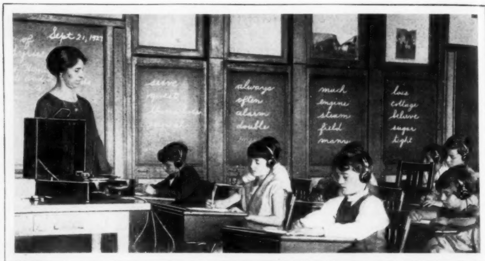
Pupils Receiving Hearing Test with Aid of Phonograph Record; Sound Is Transmitted through Headphones and Each Child Writes Down Words He Hears; Volume of Tone Can Be Varied
