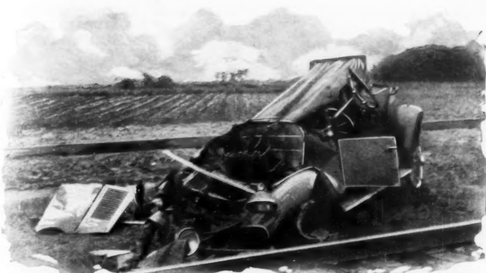
Photo by V. M. Pierce, U. S. Bureau of Public Roads
