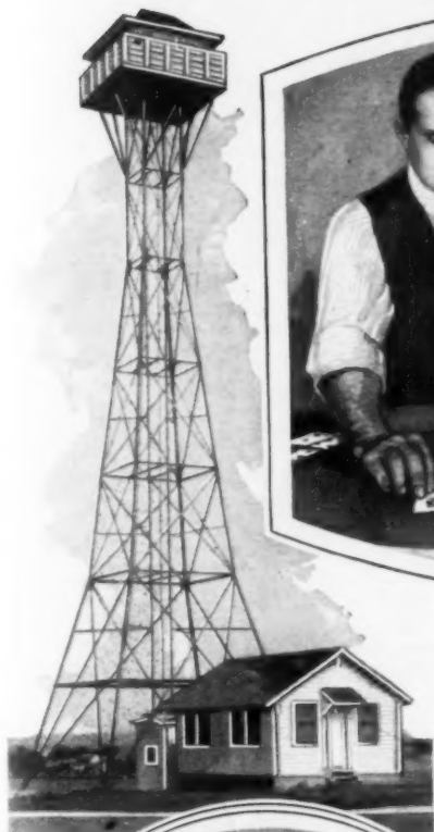
Left, Radio-Testing Laboratory Perched on Top of 125-Foot Tower Overlooking Atchison, Kans., Is Designed to Get Away from Earth Disturbances While Testing and Improving Circuits; Right, Graham McNamee and Phillips Carlin Announcing a Bridge Game
