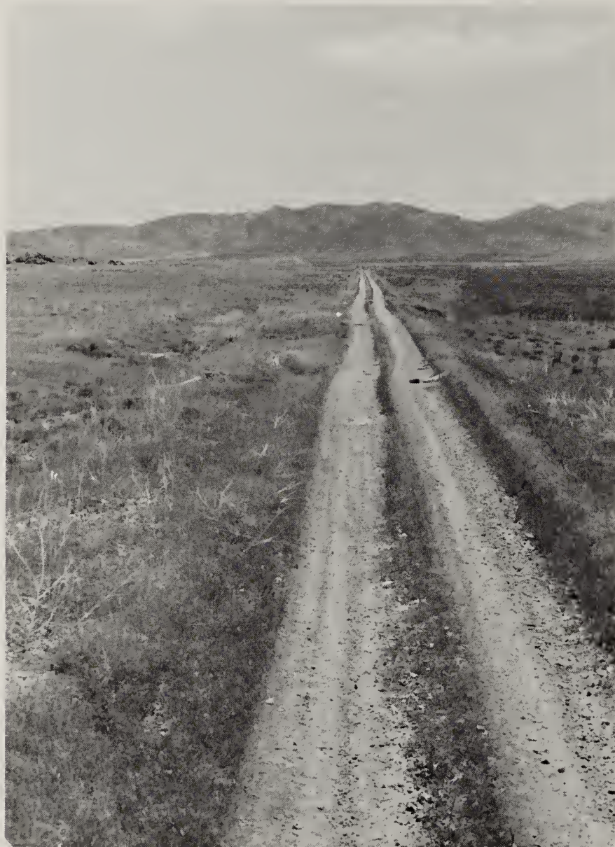
Figure 84: The siding (to the left side of photo) at Centre looking towards the east. (BLM photo)
