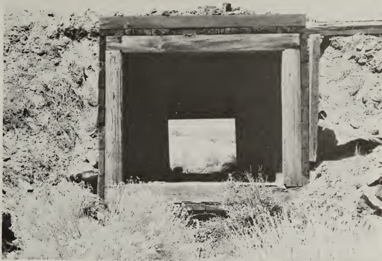
Figure 97: Wooden box culvert - about 3 feet square (BLM photo)
