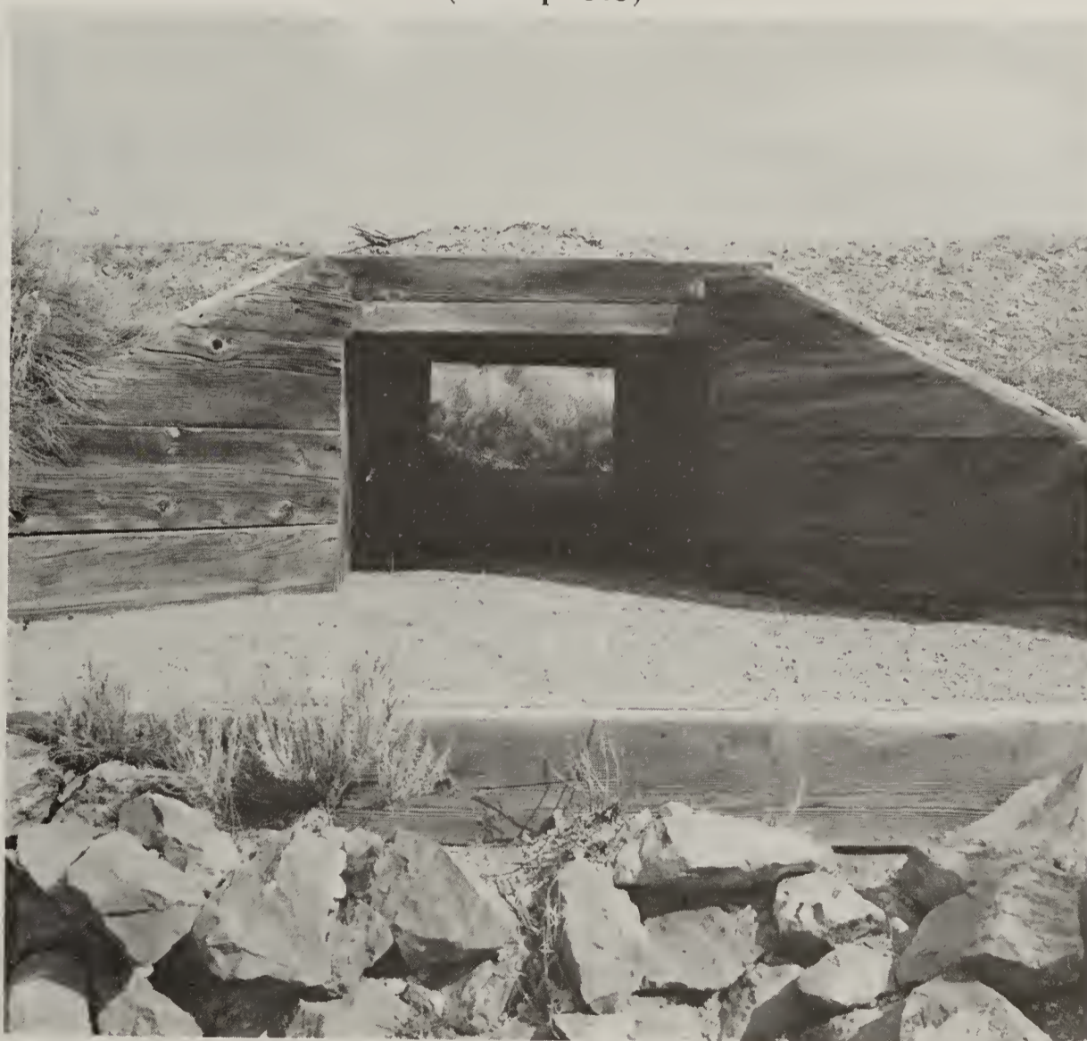
Figure 98: Wood box culvert with wing-walls, apron, and riprap. (BLM photo)
