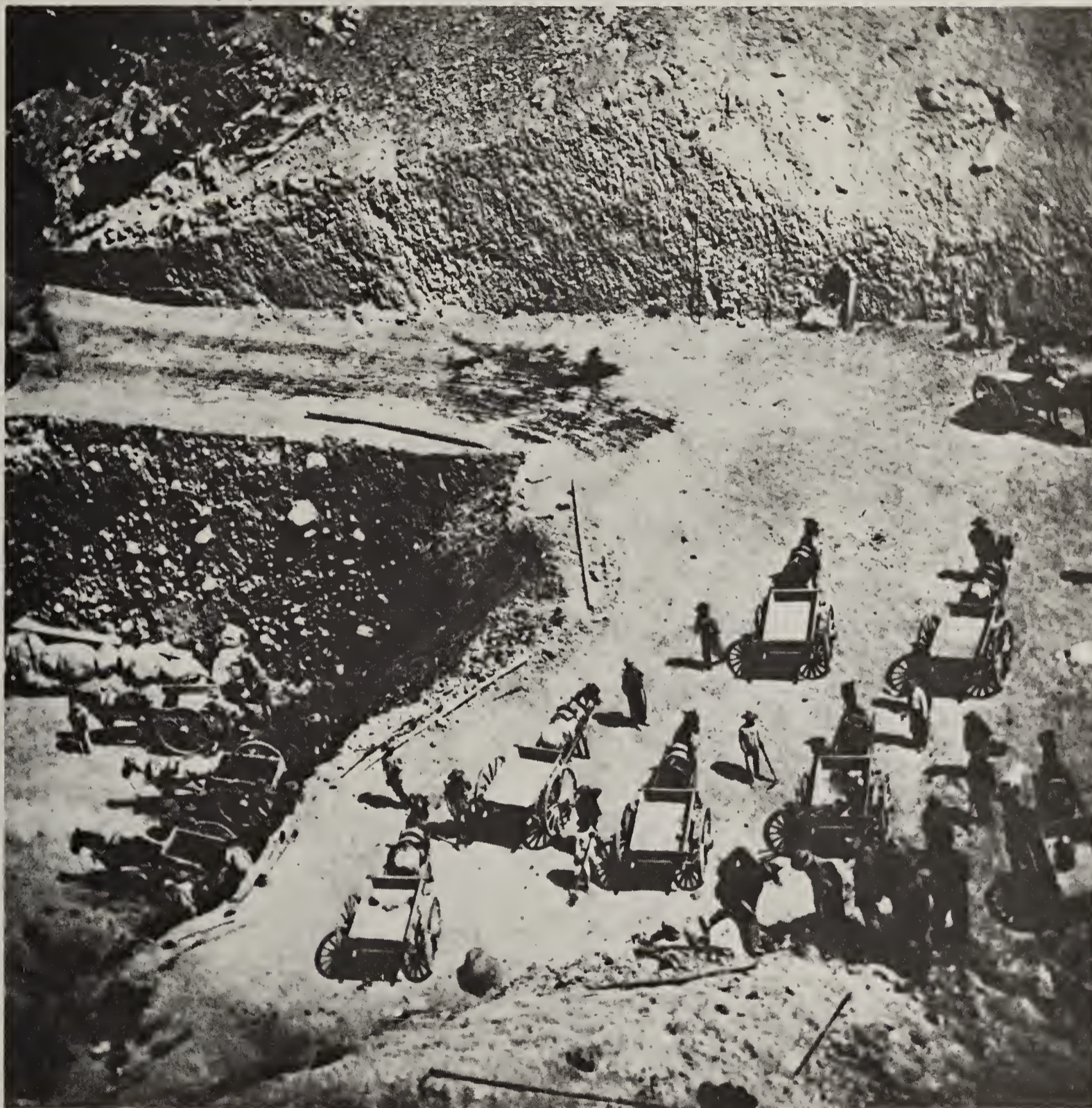
Figure 8: Chinese work gangs, horse-drawn carts, and hand tools accomplished much of the grading work (Southern Pacific, Alfred A. Hart Photograph).
