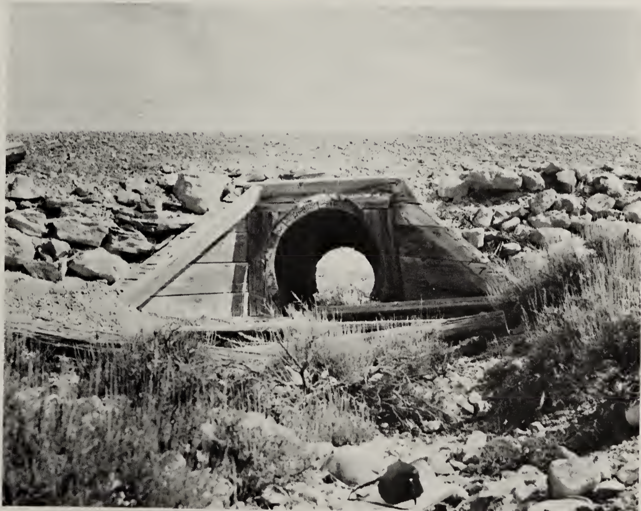
Figure 101: Wooden stave culvert with wing-walls, apron, and riprap. (BLM photo)
