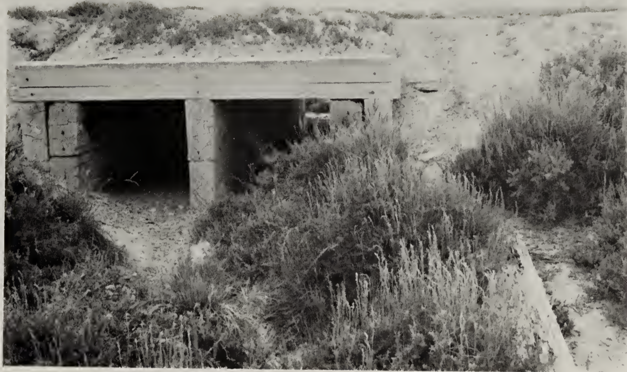
Figure 100: Dual wood box culvert (BLM photo)
