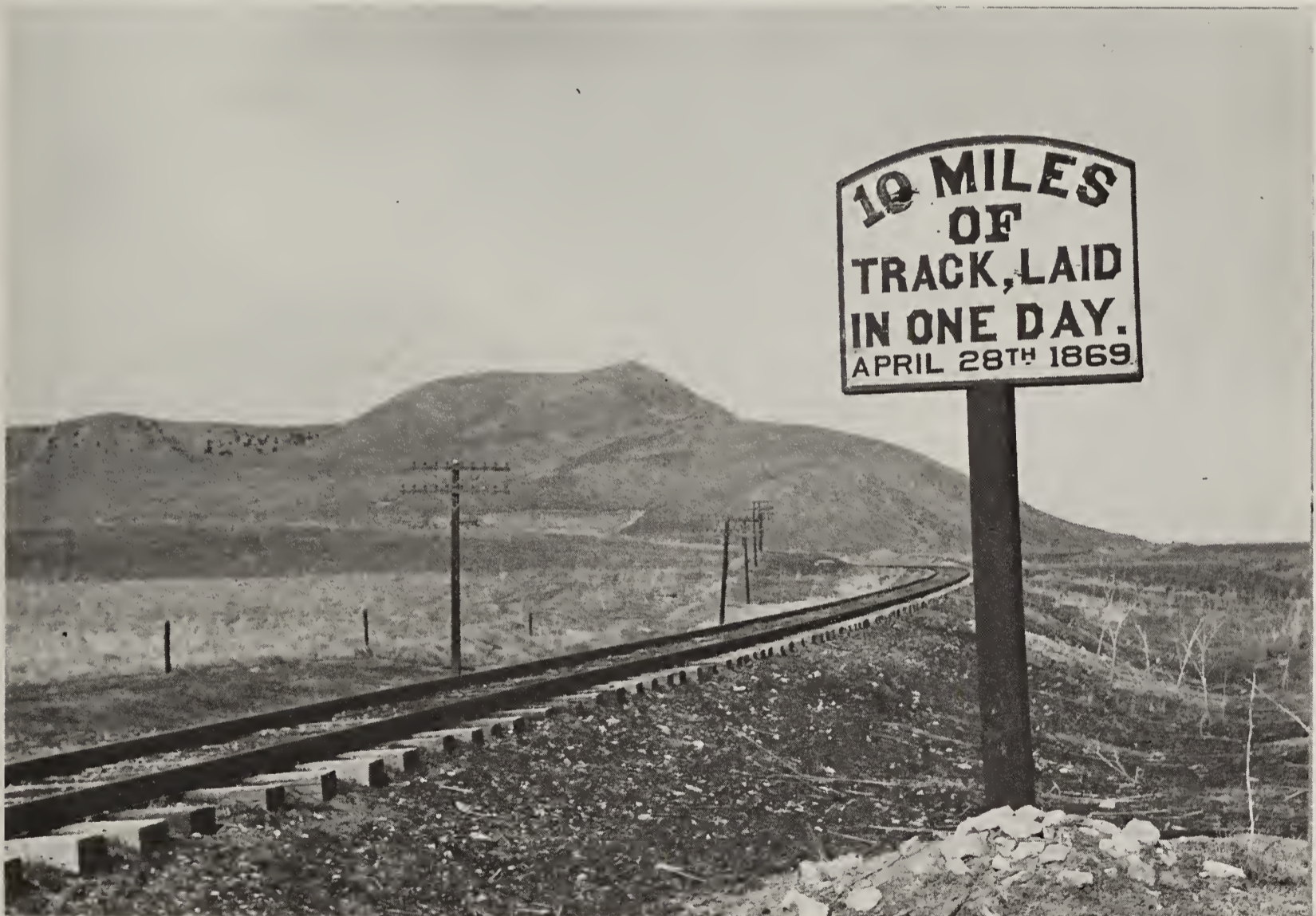
Figure 13: Ten Miles of Track Laid in One Day (Southern Pacific Photograph).
