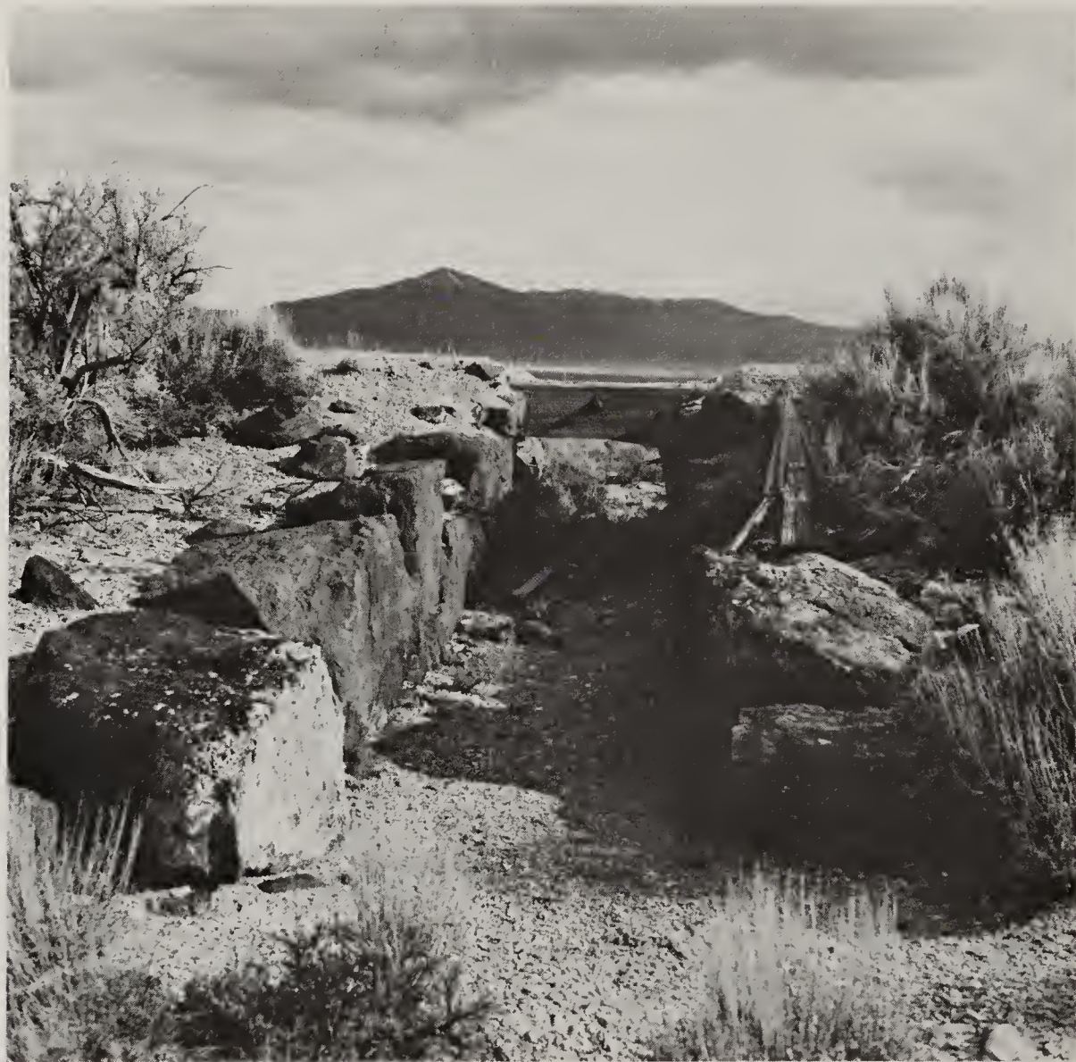
Figure 103: Open-deck stone culvert (BLM photo)
