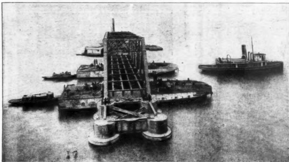
Floating Railway Span into Position
