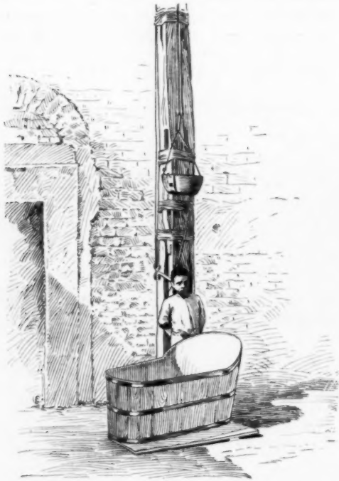
Shot is Formed in Tub of Water at Base
