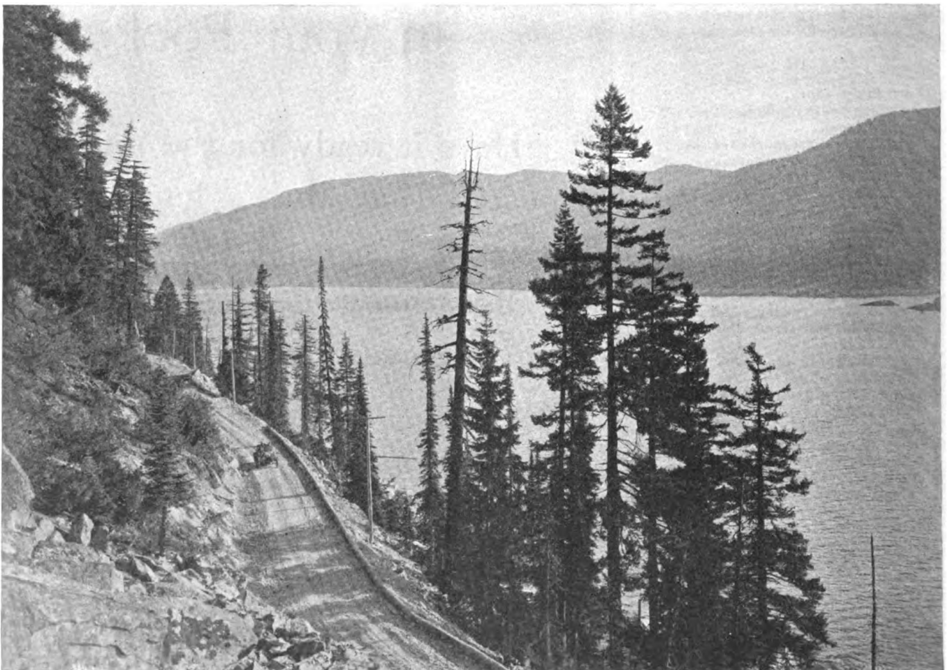
Where the new Sunset Highway across the Cascades skirts the rugged shore of Lake Ketchikan in the state of Washington
