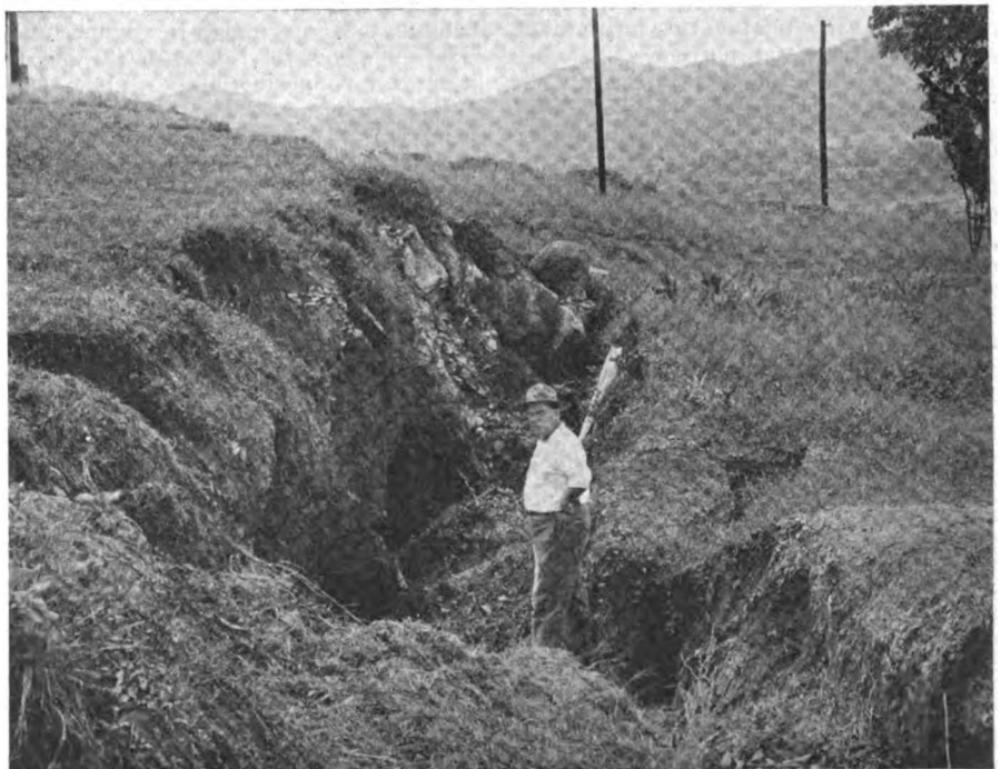
A typical crack at the outer margin of the West Culebra slide. Such cracks allow the surface water to get into and beneath the moving ground. They are the trenches of the "enemy"
