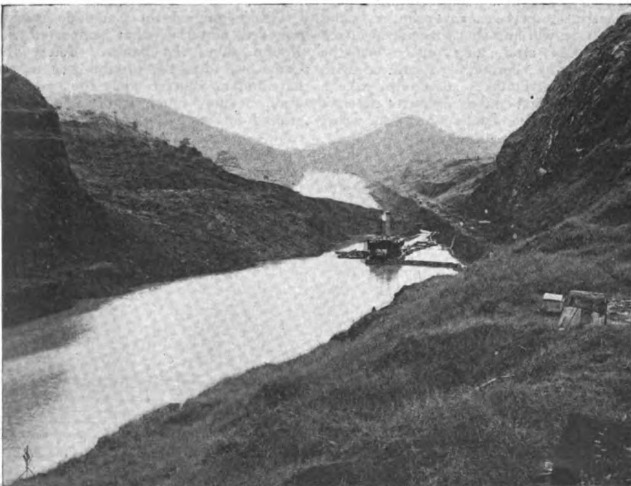
Looking southward along the Canal where it passes between Gold Hill and Contractors Hill. The Cucaracha slide completely closed the Canal channel for a distance of 2000 feet in 1914
