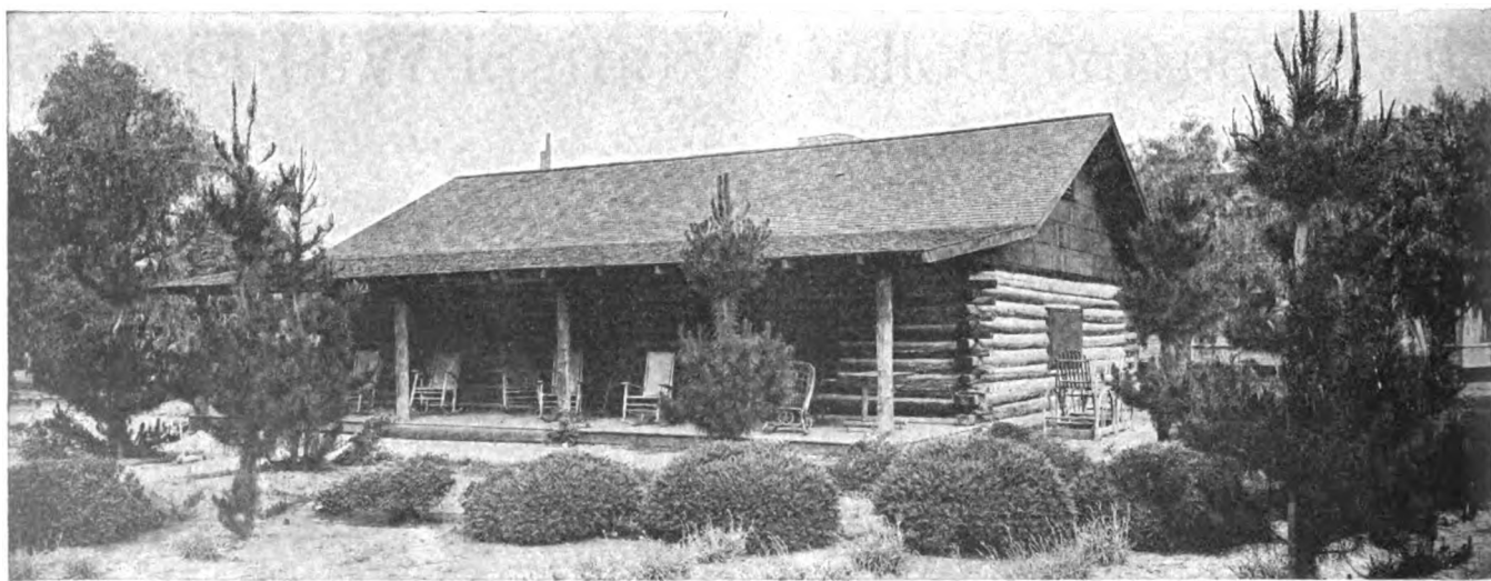
If you happen to be making a collection of houses, why not add a log cabin to the list? This one was built on the grounds of a tourist hotel and is used for informal dancing parties. It offers good suggestions for a summer camp in a forest region. A large stone chimney is in the rear wall. The interior is 24 x 34 feet
