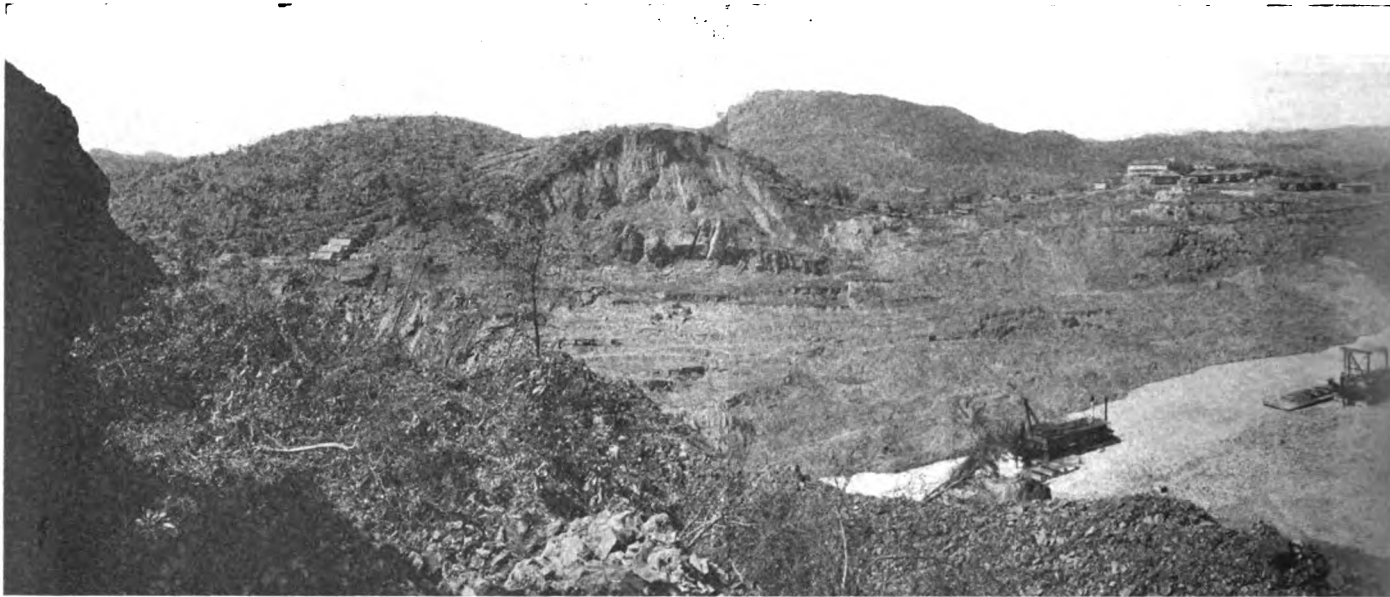
Looking northward along the Canal from the north face of Gold Hill, Dec. 21, 1915. The black mass at the left is part of Gold Hill; the trees and rocks in the foreground have fallen from its summit and from its north side. The broken hill west of the Canal is Zion Hill, a plug of basalt that has partly broken down and fallen into the West Culebra slide which involves the entire area between Zion Hill and the Canal. The houses to the right are on Culebra Hill
