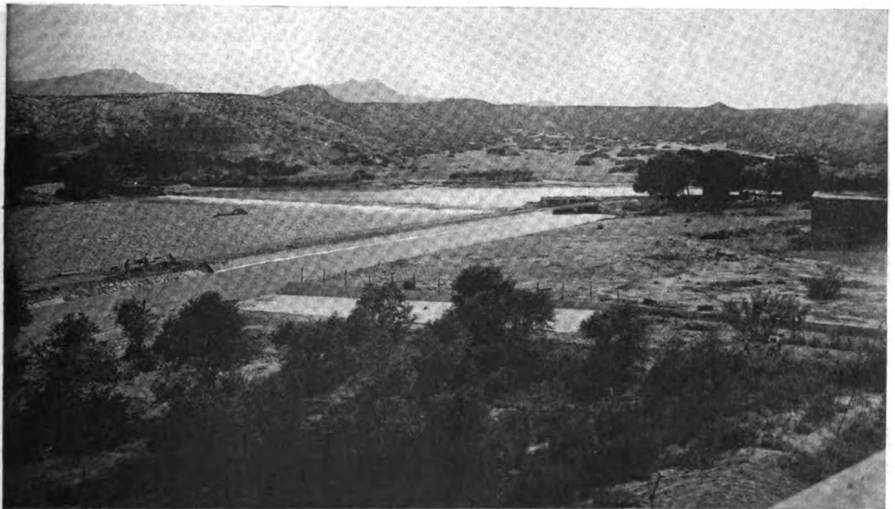
Diversion dam in the Rio Grande just above El Paso. Part of the water is delivered to Mexican irrigators on the farther side of the river, but the bulk passes through El Paso to the farmers on the American side of the Rio Grande below the capital of the Southwest
