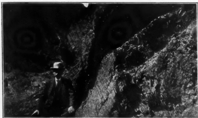
OPEN CUT OF THE USINA MINE. THE BEDDED ROCKS AT RIGHT ARE SCHISTOSE SPECULAR IRON
