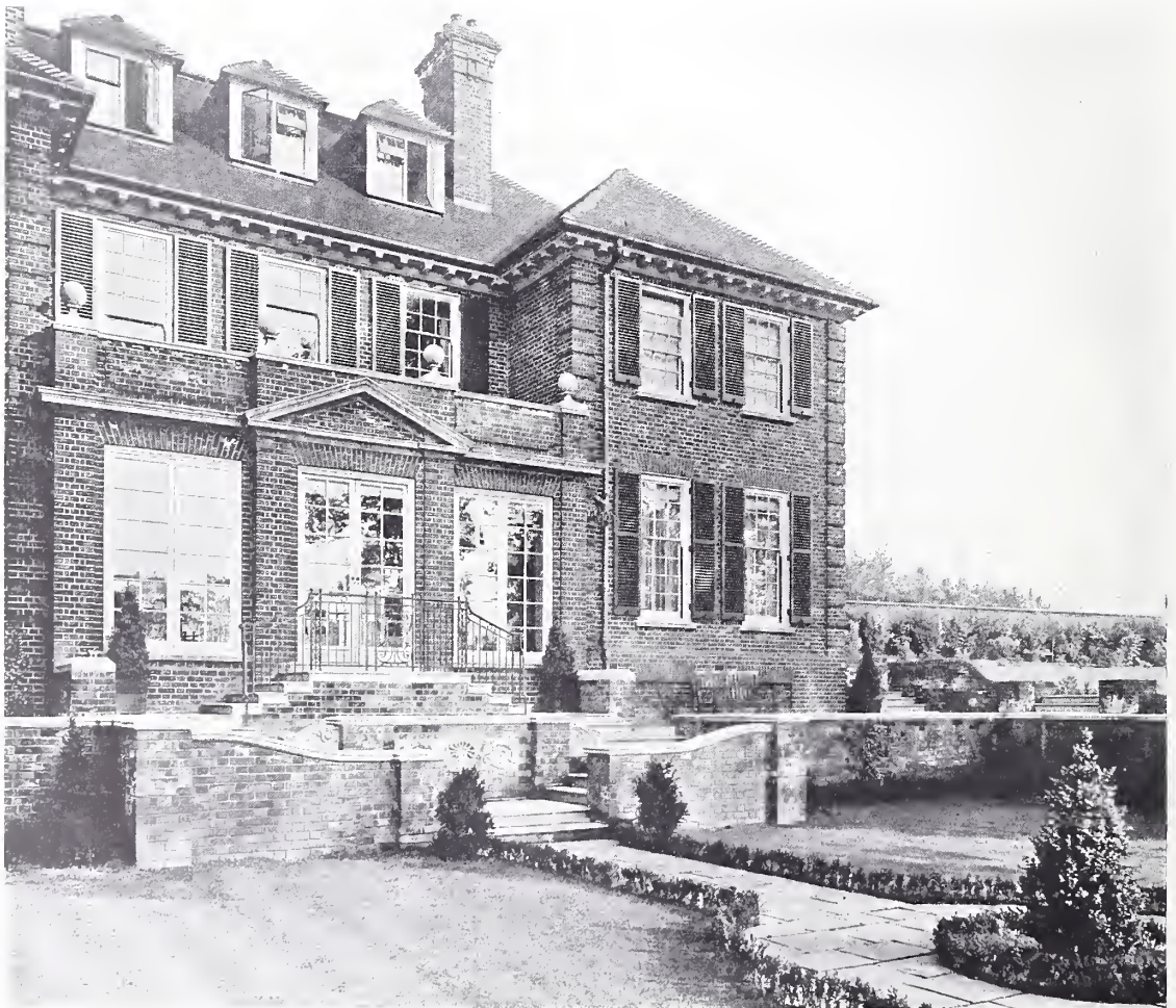
TEMPLEHILL HOUSE, HAMPSTEAD
