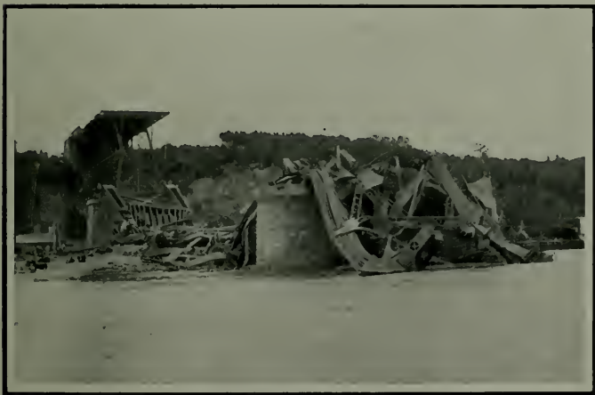
THE QUEBEC BRIDGE AFTER THE ACCIDENT
