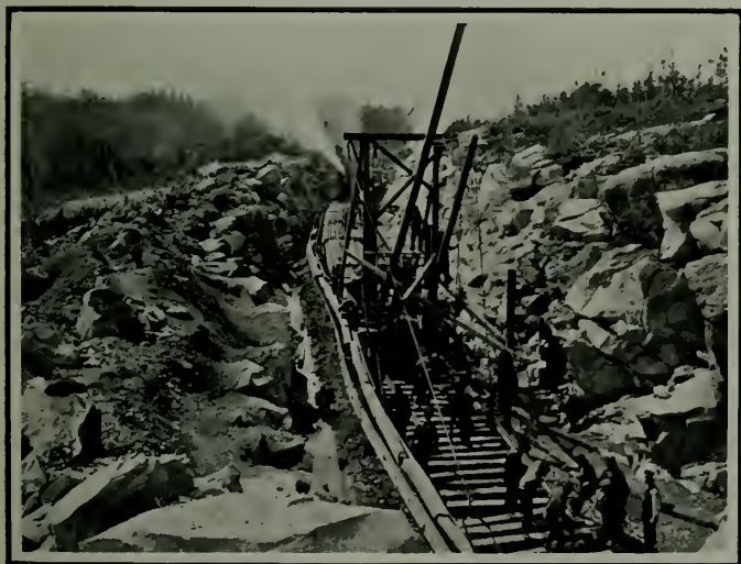
LAYING THREE MILES OF METALS PER DAY
