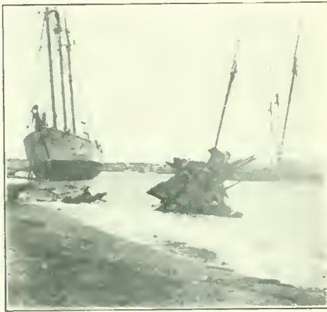
After the blow was over.
