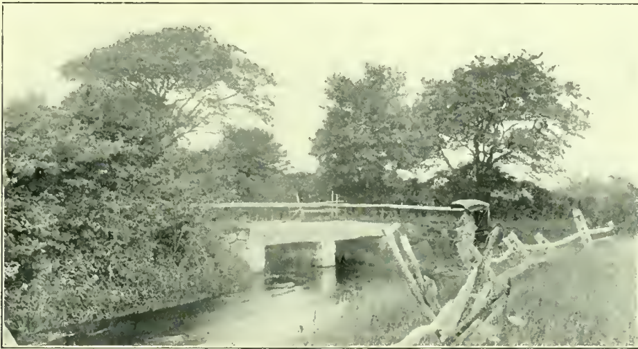
The State Road crosses Mill Brook.
