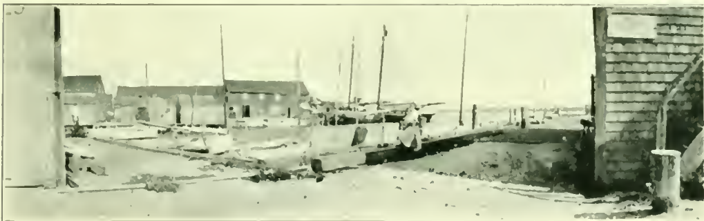
Edgartown's docking facilities.
