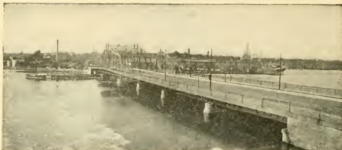
NEW BEDFORD AND THE FAIRHAVEN BRIDGE
