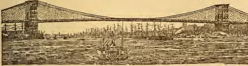
New York and Brooklyn Suspension Bridge: total length, 5,989 ft.; river span, 1,595.5 ft.; completed in 1883.
