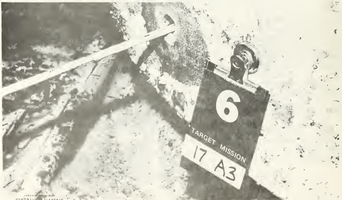
FIGURE 19. Impact Six, Target 17, Perforation of Right Side of Turret.
