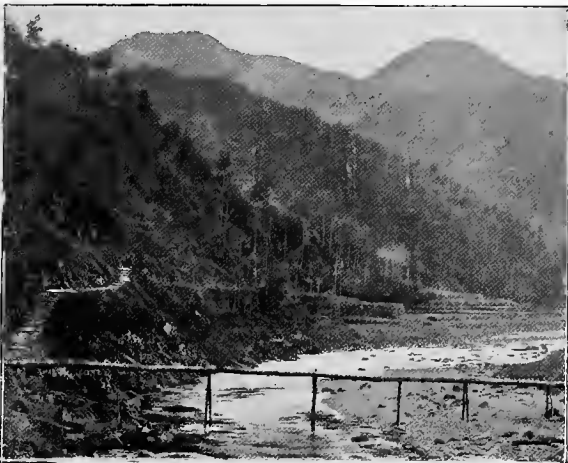
BAMBOO BRIDGE ERECTED AS WORK OF MERIT.
