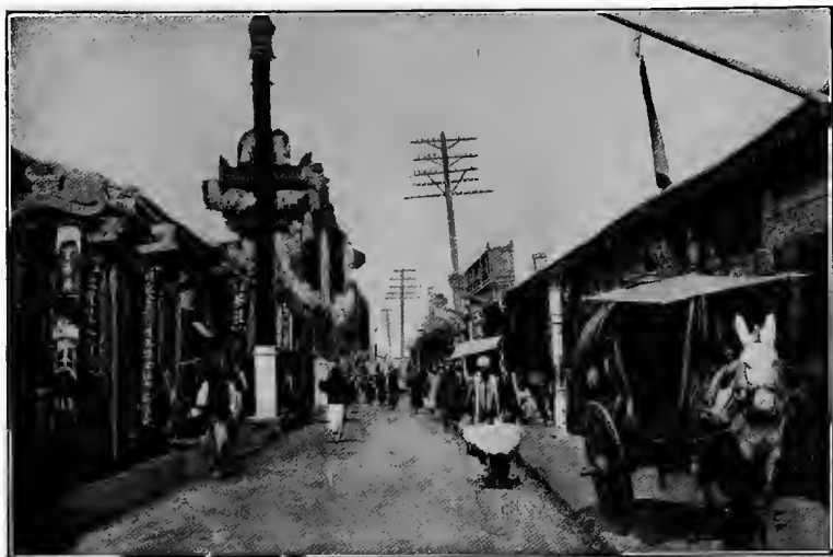
MAIN STREET, NEWCHWANG : COVERED CART AND HANDSOME SHOP SIGNS.
