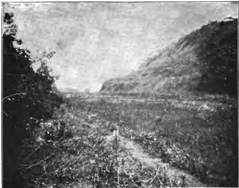
FIG. 1.—THE EXCAVATION OF THE BOHIO LOCK SITE.
