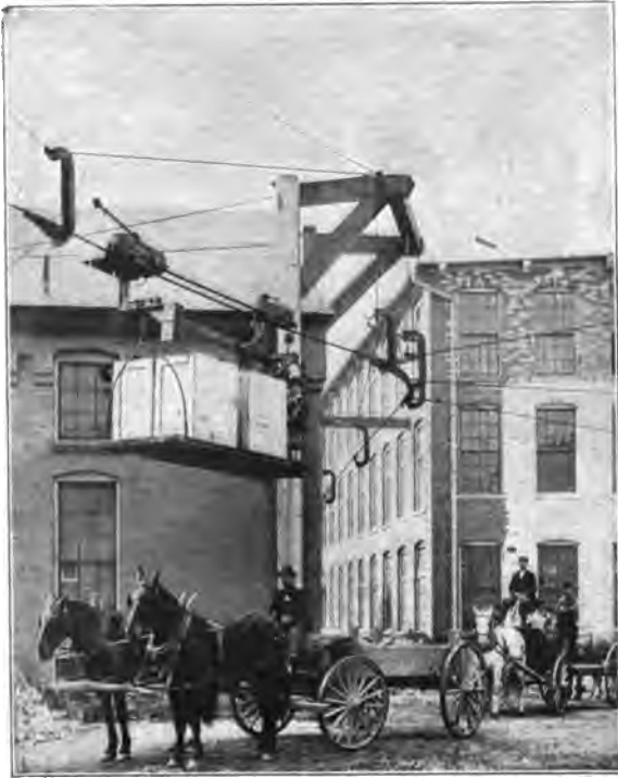
FIG. 1.—CURVE CONSTRUCTION OF CABLE TRACK WITH HEAVY LOAD.
