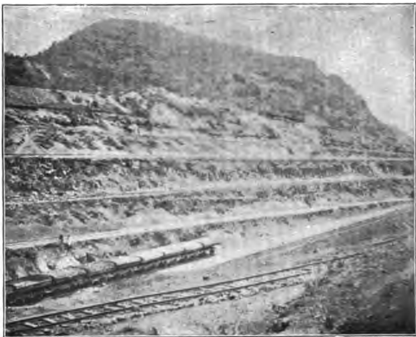
FIG. 2.—THE EASTERN FACE OF THE CULEBRA CUT.
