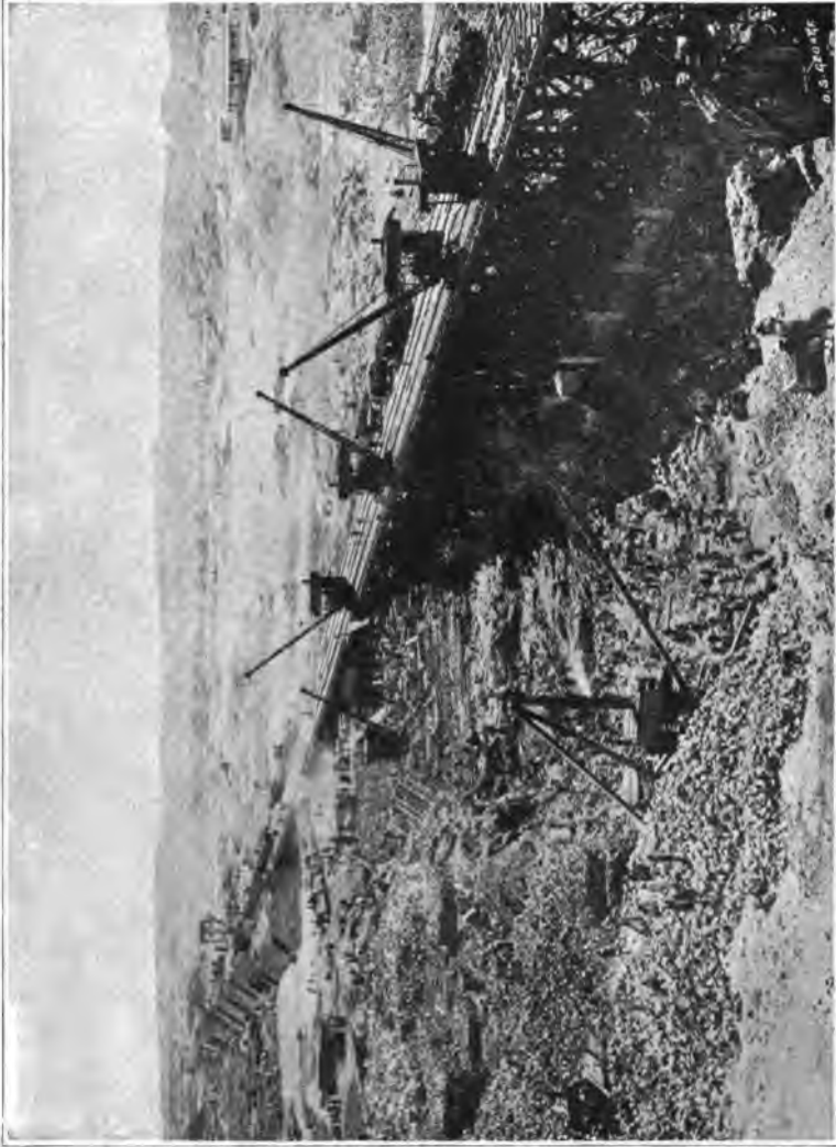
THE ASSUAN DAM IN COURSE OF CONSTRUCTION—FILLING IN THE EXCAVATIONS WITH MASONRY.
