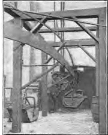
FIG. 2.—BUCKETS FILLED FROM CHUTES.
