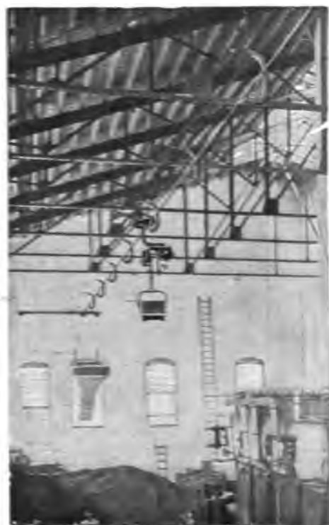
CABLE CONSTRUCTION WITH TELPHER, ELECTRIC HOIST, AND BUCKET.
