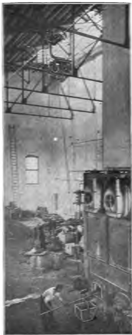
CABLE CONSTRUCTION WITH TELPHER, ELECTRIC HOIST, AND BUCKET.
