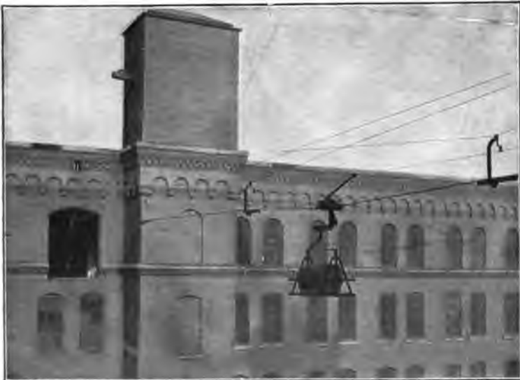
FIG. 2.—CABLE CONSTRUCTION, LINE 97 FEET FROM GROUND, ILLUSTRATING SUSPENSION CABLE, TRACK CABLE, AND HANGERS.
