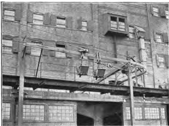
FIG. 3.—SOLID RAIL COMBINED WITH CABLE CONSTRUCTION
