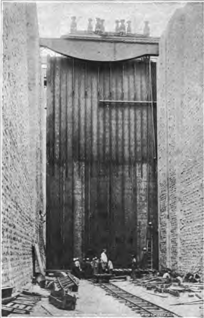
LOCK GATE ON THE SHIP CANAL AROUND THE DAM, BUILT FROM DESIGNS MADE FOR THE NICARAGUA CANAL.
