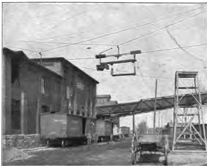
FIG. 1.—TELPHER, TRAILER, ELECTRIC HOIST, WITH PLATFORM CARRIER.
