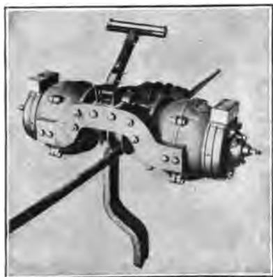
FIG. 1.—CENTER-BEARING TELPHER.
