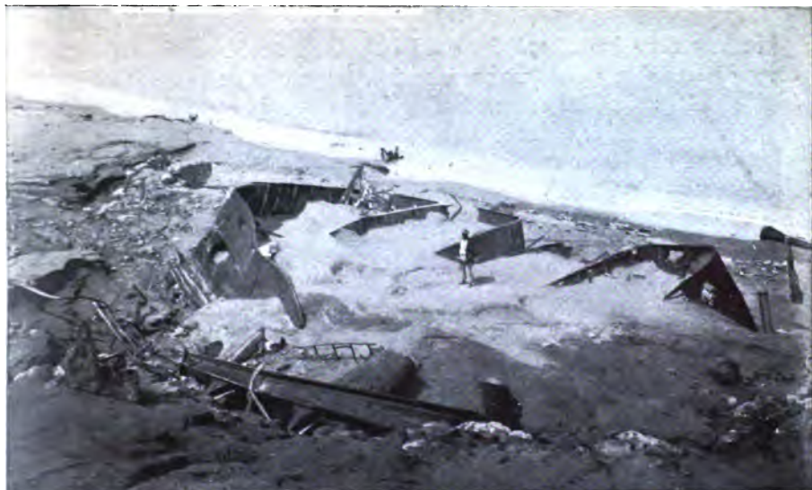
FIG. 1.—ST. PIERRE. RUINS OF THE GREAT DISTILLERY IN THE FORT QUARTER OF THE CITY, SHOWING HOLES IN THE IRON TANKS DUE TO VOLCANIC BOMBARDMENT.
