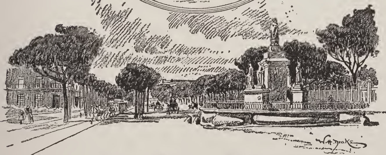
Street Scene, Havana. (The drive of Carlos III)
