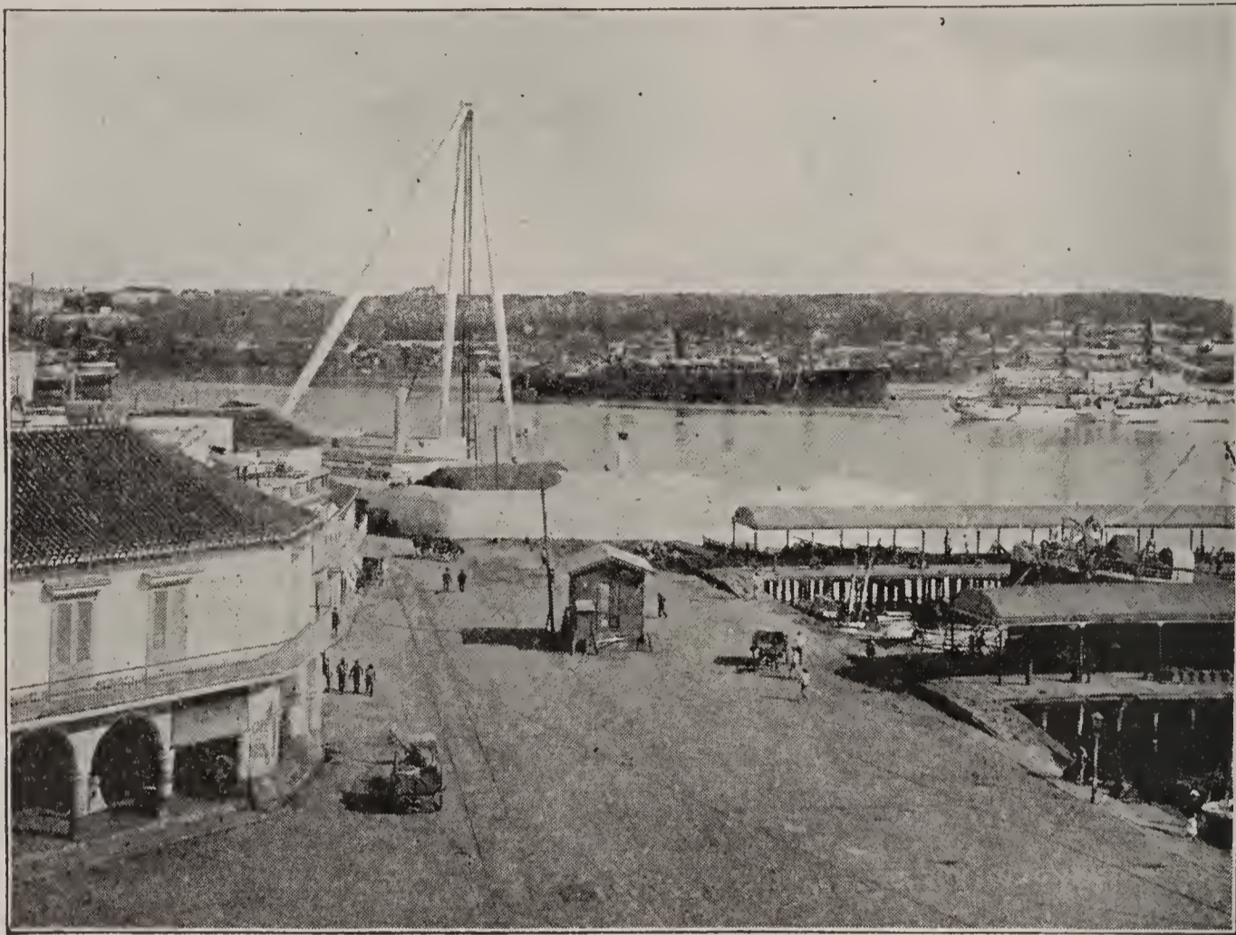
NAVAL CRANE AT HAVANA
