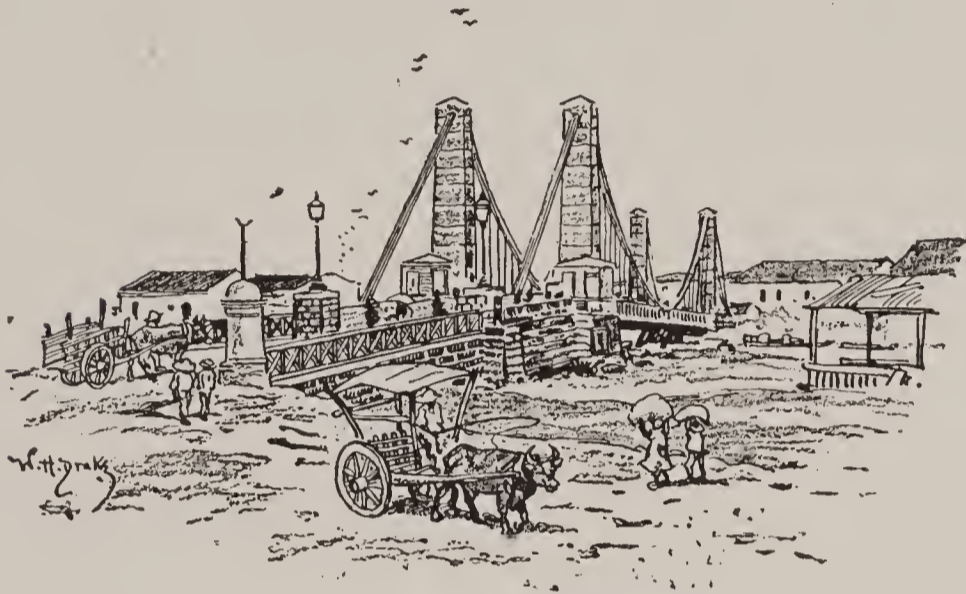
Iron Suspension Bridge over Pasig River Manila.
