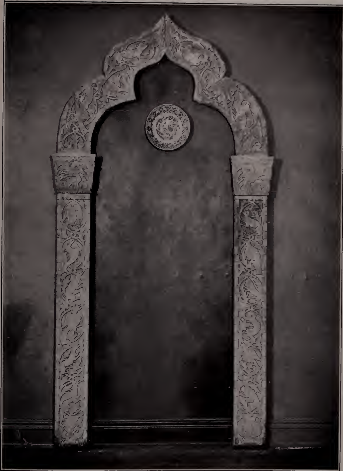
VENETIAN STONE DOORWAY WITH BYZANTINE DETAIL.
