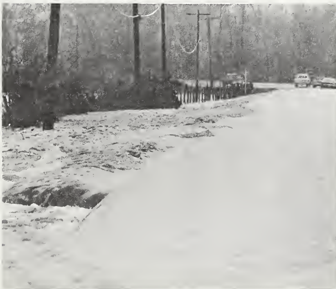
This road was flooded by Burcham Creek near Cloverdale in March of 1973. Note the erosion of the shoulders in the lower left-hand corner.
