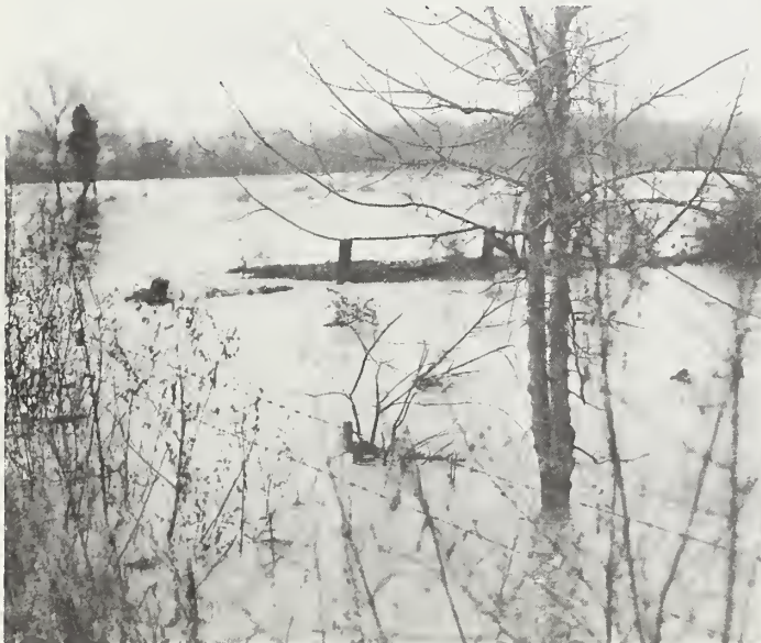
Floodwater on Cypress Creek looking upstream from Cloverdale-Threet Road.
