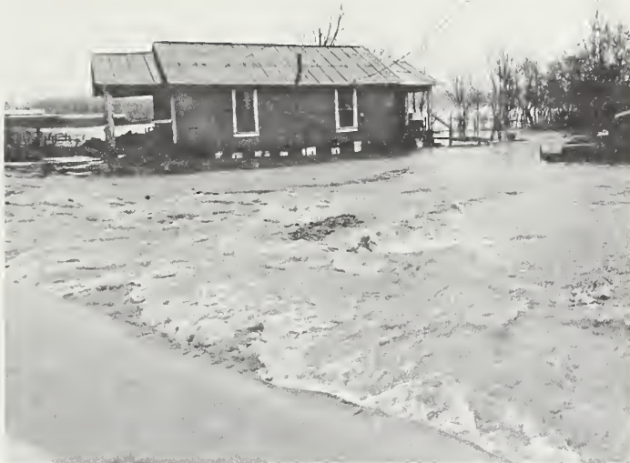
Flooding of this house and adjoining land was caused by Burcham Creek near Cloverdale in March of 1973.
