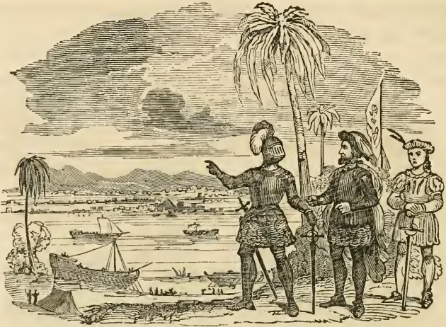
Cortez building Brigantines on the Lakes.
