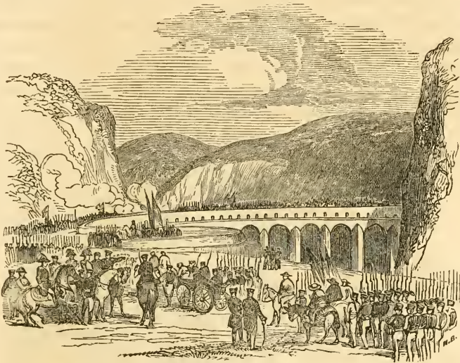
The Army crossing the National Bridge near Cerro Gordo.
