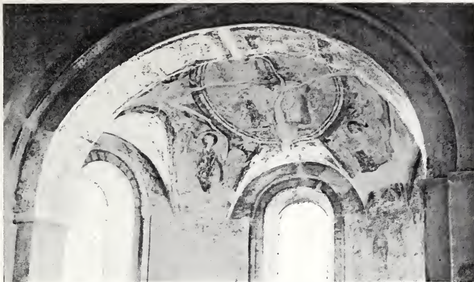
COPFORD CHURCH. CONDITION OF FRESCO BEFORE RESTORATION. (SEE PLATE CXC.)
