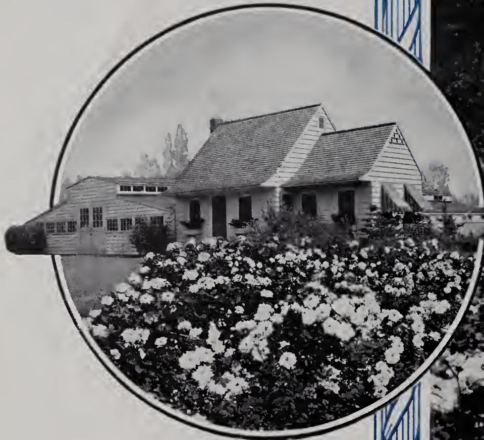
Office with section of the huge shed in background
