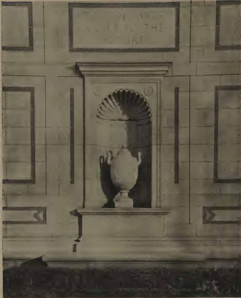
Detail of Dudley Allen Memorial Art Building
