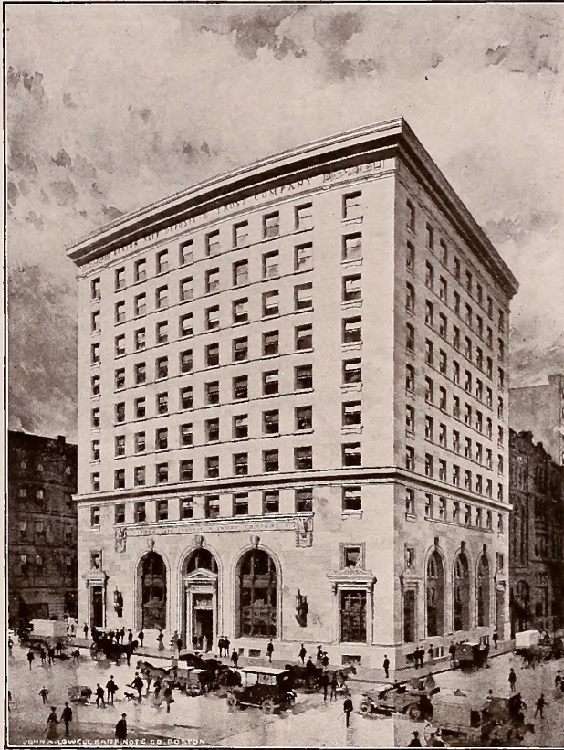
BOSTON SAFE DEPOSIT & TRUST CO. BUILDING Devonshire, Arch and Franklin Streets, Boston
