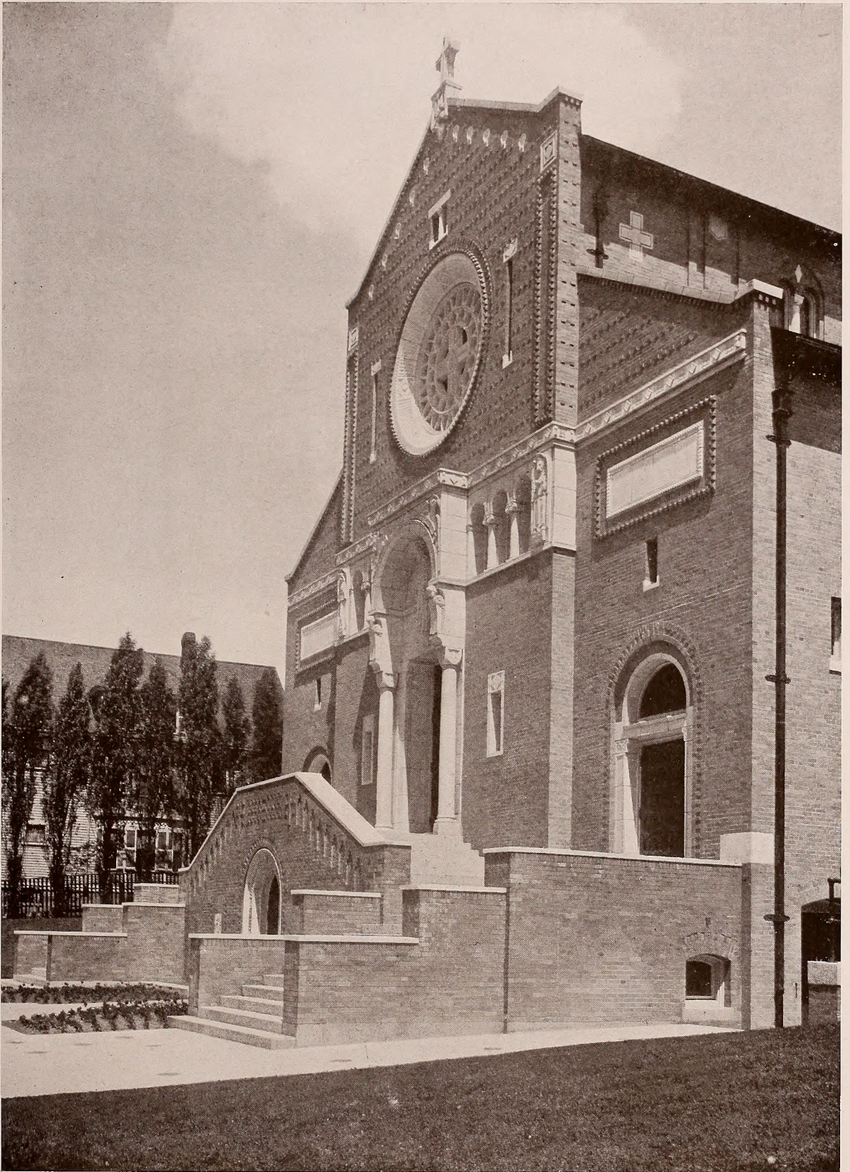
CHURCH IN SOMERVILLE, MASS. Maginnis & Walsh, Architects
