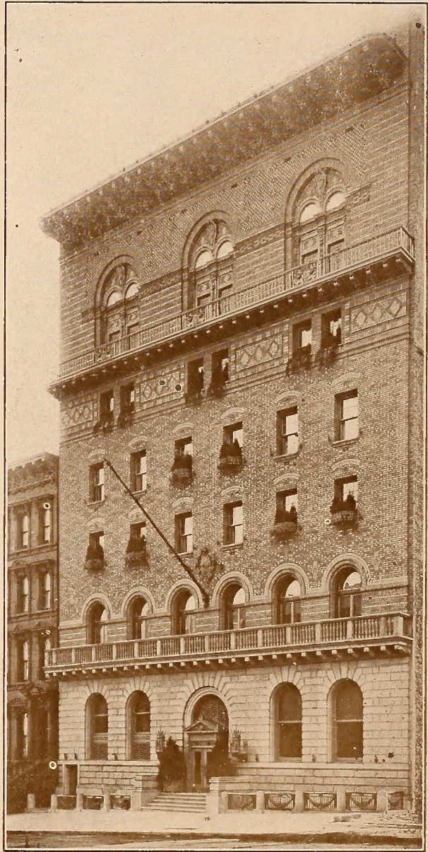
LOTOS CLUB, WEST 57TH STREET, NEW YORK. Donn Barber, Architect.
