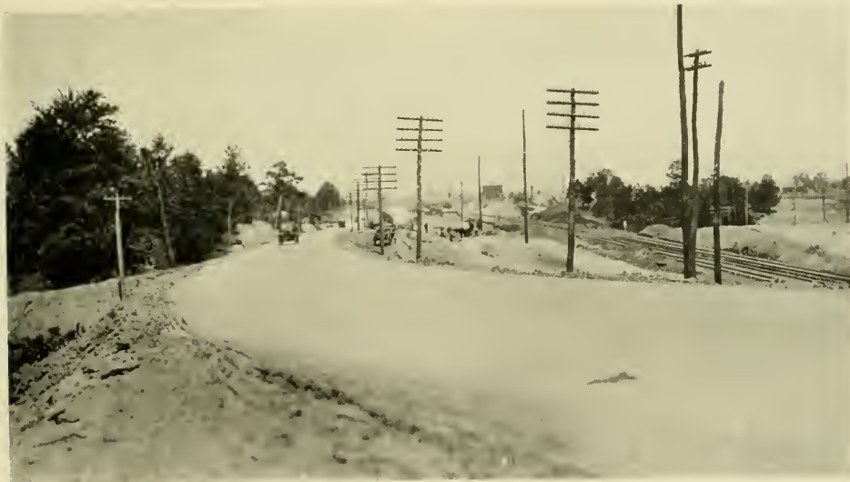
14. CONCRETE ROAD, CAMP SEVIER, GREENVILLE, S. C.
