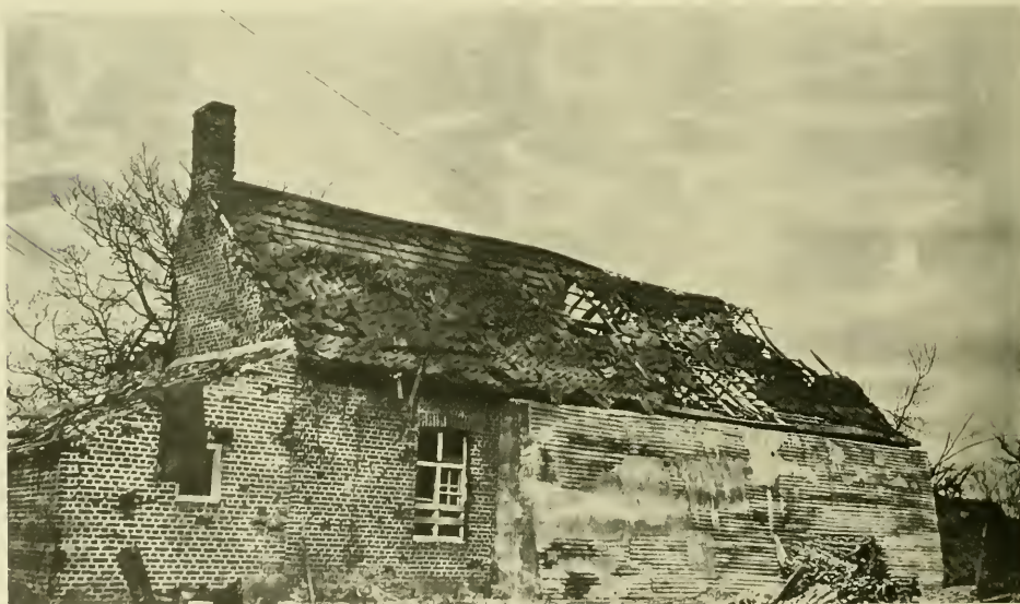
47. LIGHT RAILWAY CONTROL STATION, PIONEER JUNCTION, CANAL SECTOR, BELGIUM
