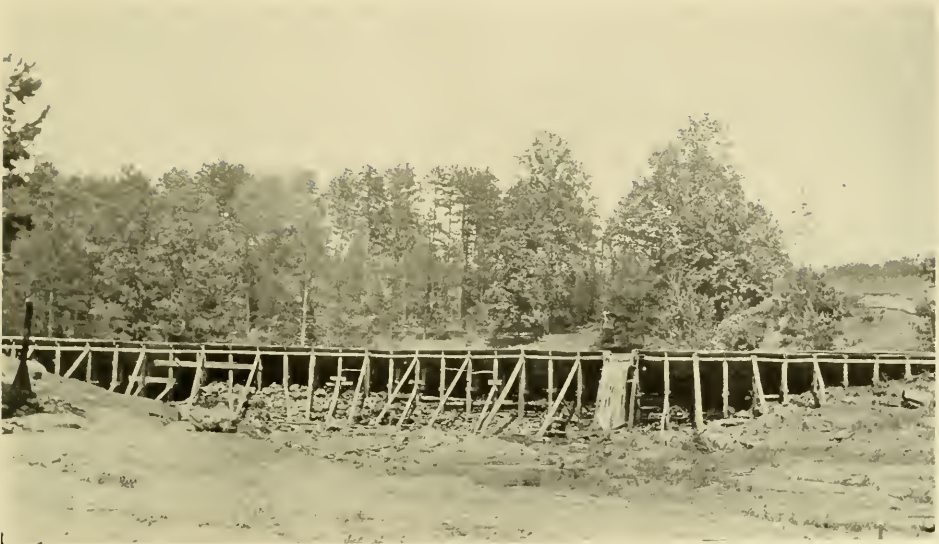
9. JONES' POND DAM, CAMP SEVIER, GREENVILLE, S. C.
