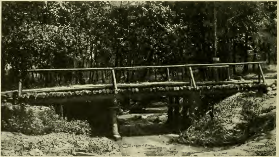
16. BRIDGE, CAMP SEVIER, GREENVILLE, S. C.
