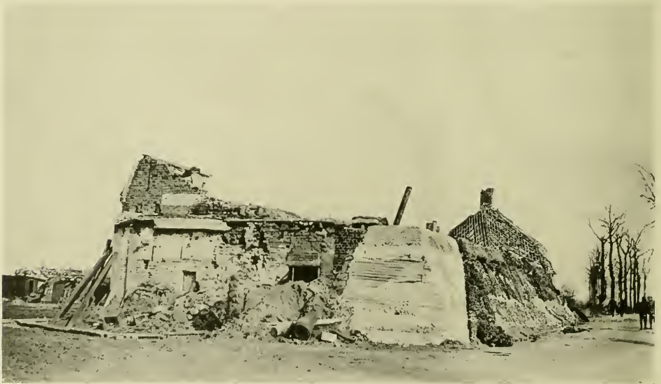
39. BELGIAN BATTERY CORNER FIRST AID DRESSING STATION, CANAL SECTOR, BELGIUM
