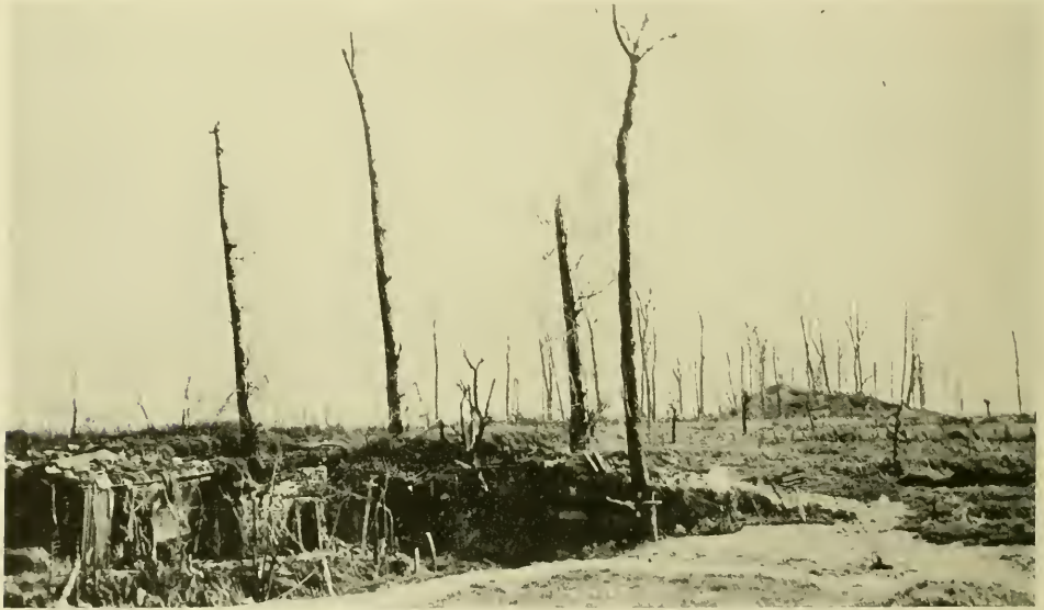
51. RT. BATTALION HEADQUARTERS AT WHITEHOUSE, CANAL SECTOR, BELGIUM, AUGUST, 1918
