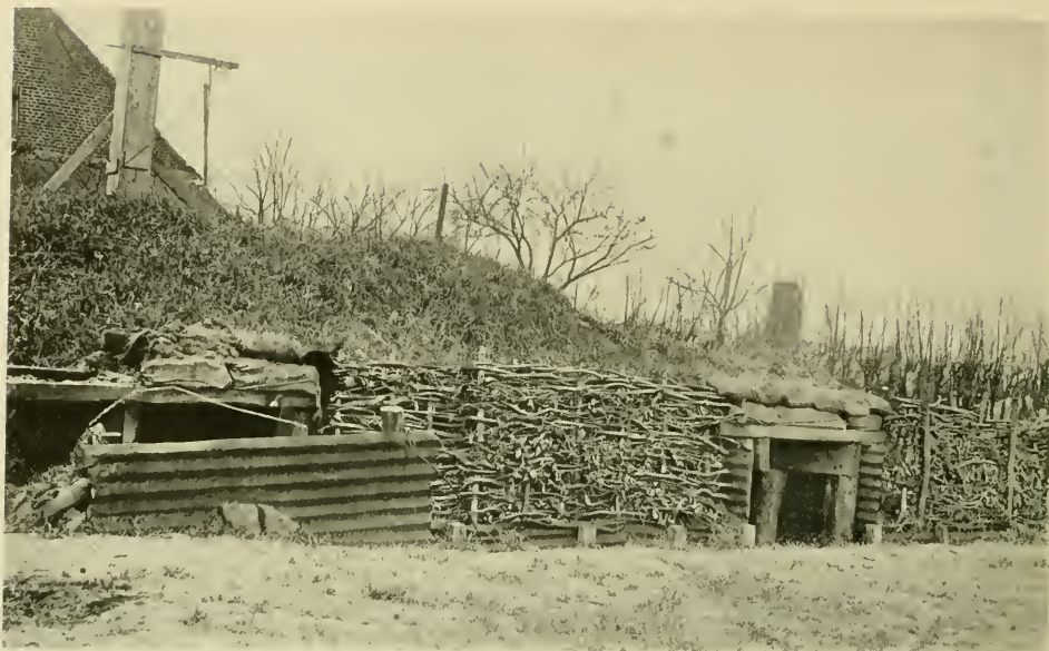
29. A "CLOSE-UP" OF A PYRAMID SHELTER, BRANDHOEK LINE, CANAL SECTOR
