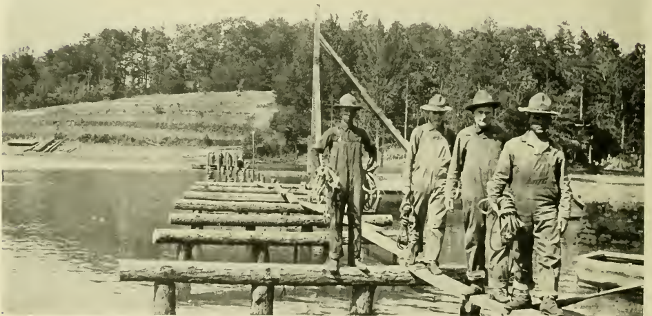
12. CONSTRUCTING PILE BRIDGE, JONES' POND, CAMP SEVIER, GREENVILLE, S. C.
