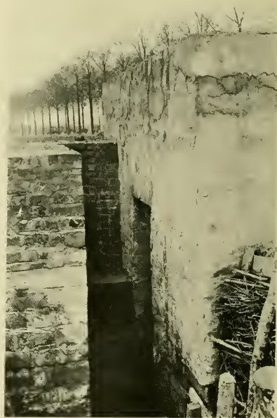
31. A CONCRETE BLOCK MACHINE-GUN PILL-BOX, CANAL SECTOR, BELGIUM
