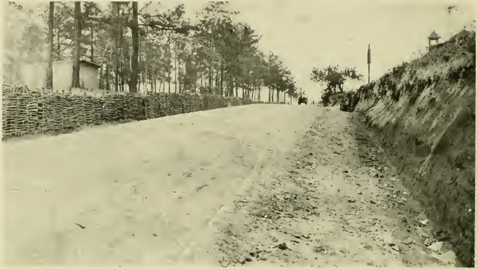
15. SAND CLAY ROAD, LEFT BANK REVETTED WITH HURDLES, CAMP SEVIER, GREENVILLE, S. C.
