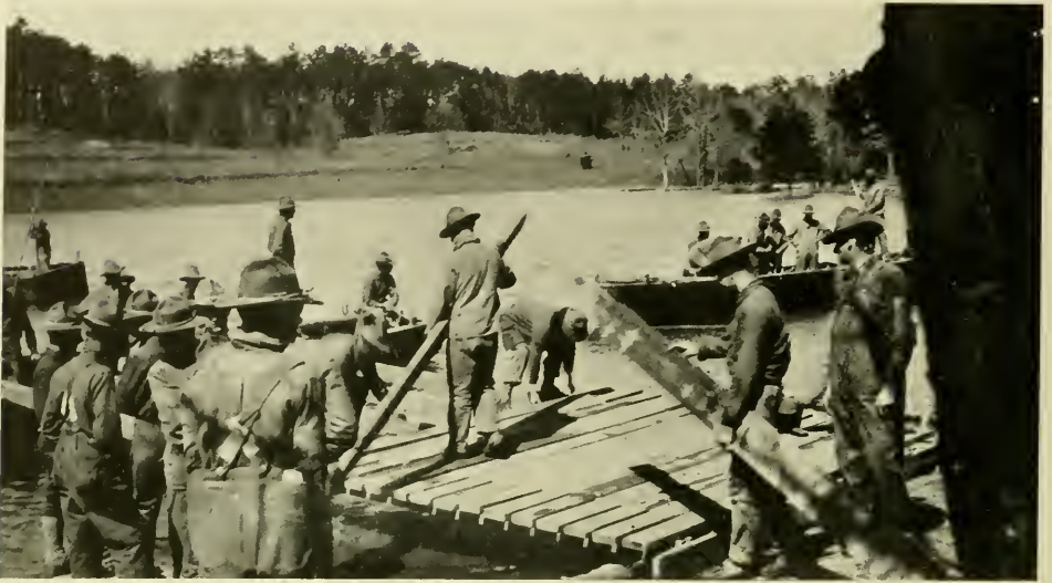
11. CONSTRUCTING PONTOON BRIDGE, JONES' POND, CAMP SEVIER, GREENVILLE, S. C.
