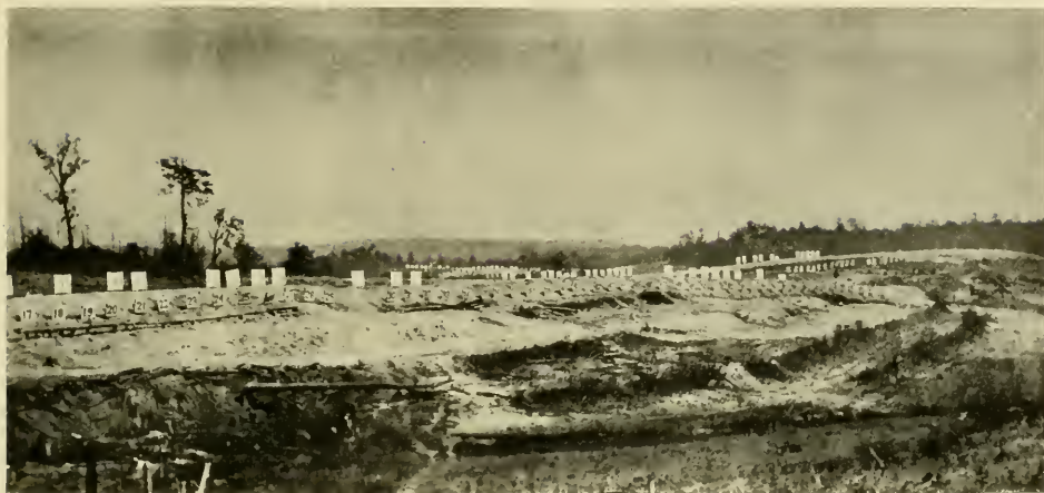
1. DIVISION RIFLE RANGES, CAMP SEVIER, GREENVILLE, S. C. Laid out and constructed under supervision of the 105th Engineers
