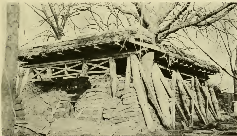
41. TYPE OF BOMB-PROOF SHELTERS, CANAL SECTOR, BELGIUM
