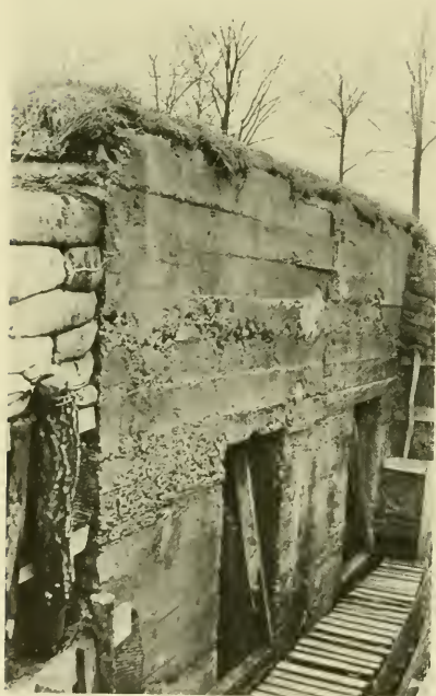
30. A MONOLITHIC CONCRETE MACHINE-GUN PILL-BOX, CANAL SECTOR, BELGIUM
