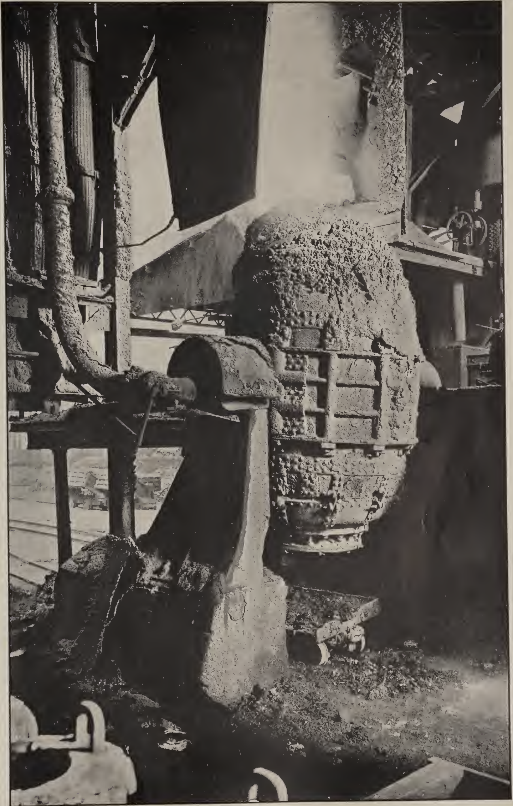
BESSEMER CONVERTER BLOWING A HEAT OF STEEL
