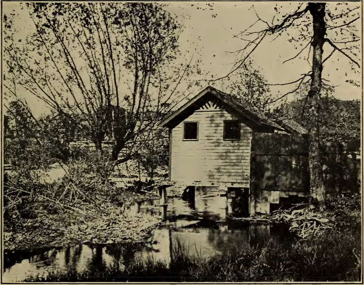
FIG. 18.—THE OVERHANGING PRIVY.
