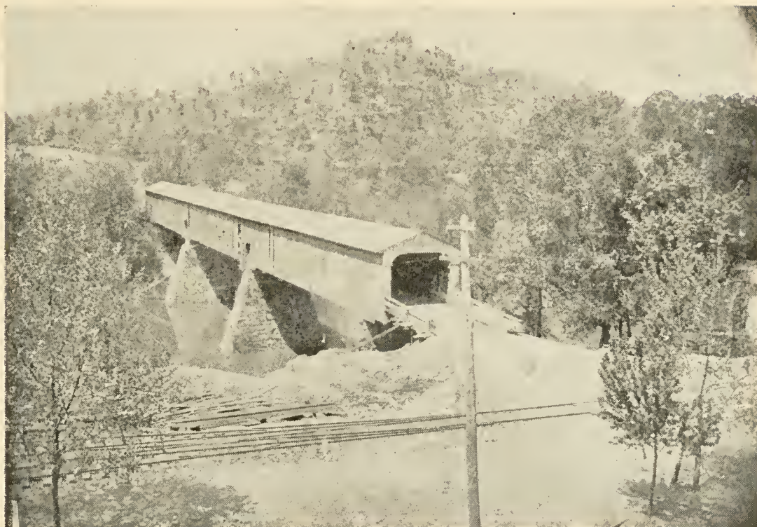
THE OLD BROAD STREET BRIDGE OVER THE ETOWAH RIVER.
