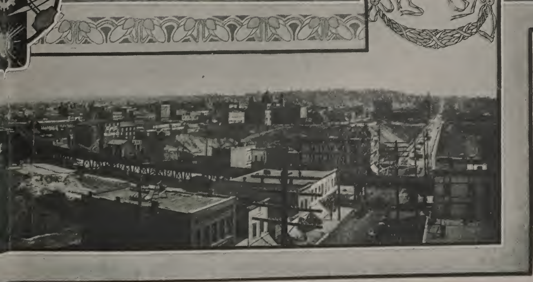
water. At extreme low water this fall of 68 feet develops 15,000 electrical horsepower. The Spokane e view of Middle Falls and manufacturing district, taken in 1906. Electrical power amous silver-lead mines of the Coeur d'Alenes, Idaho, which produce ual lead output of the world.
