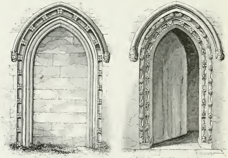
Doorways. Kislisbury. Northants. c 1330
