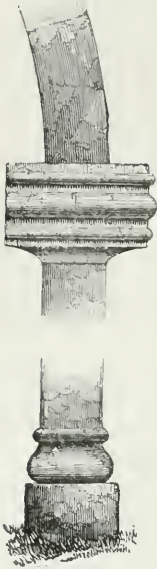
Corhampton Doorway. Impost and Base.
