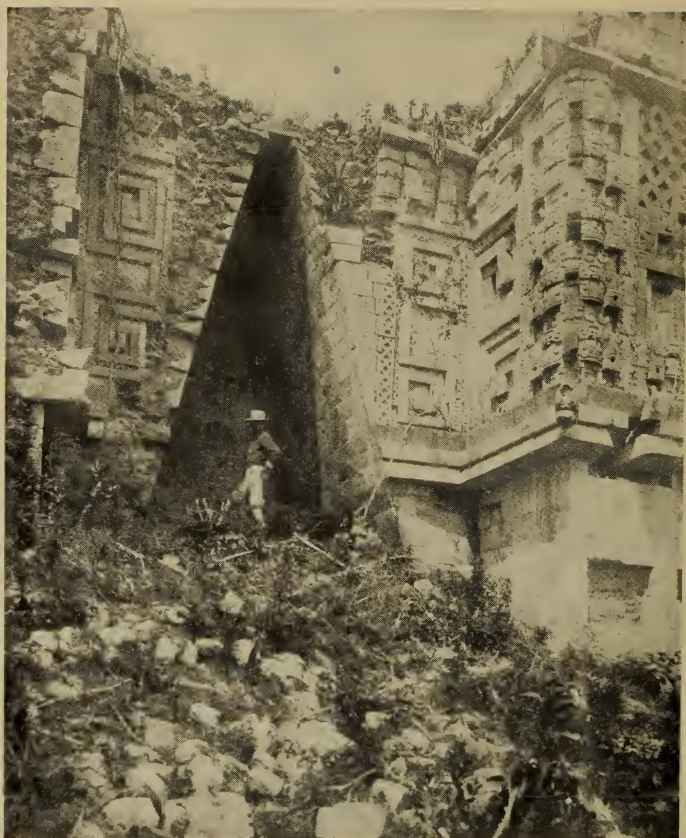
Plate XVII. A Sealed Portal Vault in the House of the Governor at Uxmal, a Building of the Second Empire, probably Thirteenth Century. The venter character of the cut stone comes out clearly. Peabody Museum photograph.
