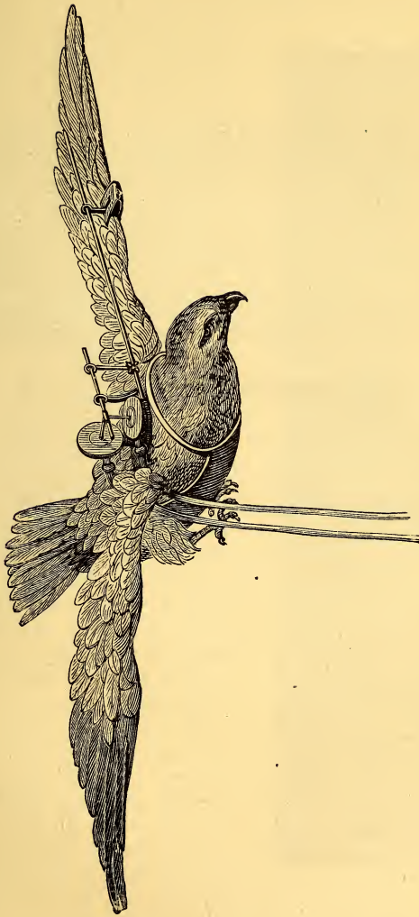
FIG. 99.—Buzzard flying with the apparatus which gives the signal of the movements described by the extremity of its wing.
