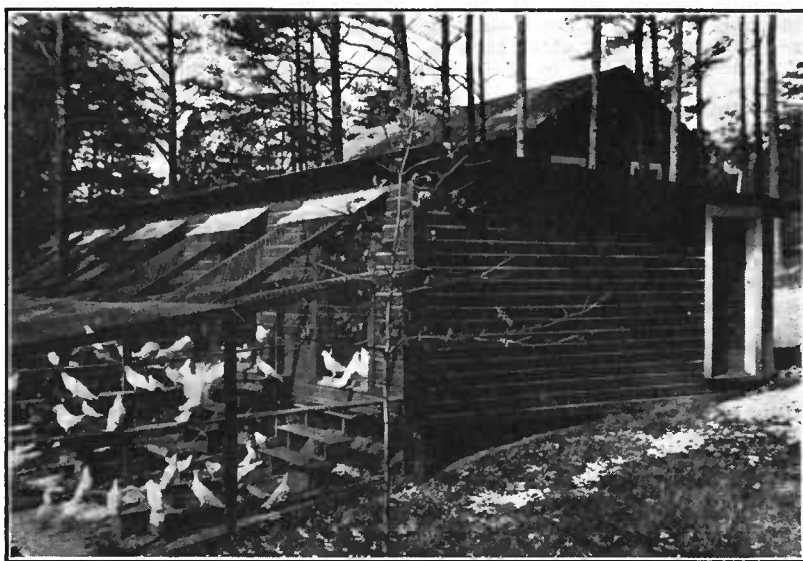
Fig. 8.—Shed-roof pigeon house with partly open front. Attached fly contains a concrete bathing and drinking basin supplied with running water
