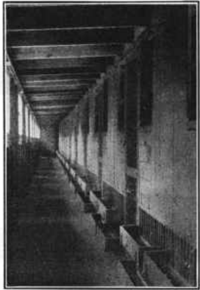
FIG. 12.—Alley in rear of pigeon house, showing arrangement of feed hoppers
