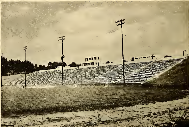
Burlington High School Stadium
