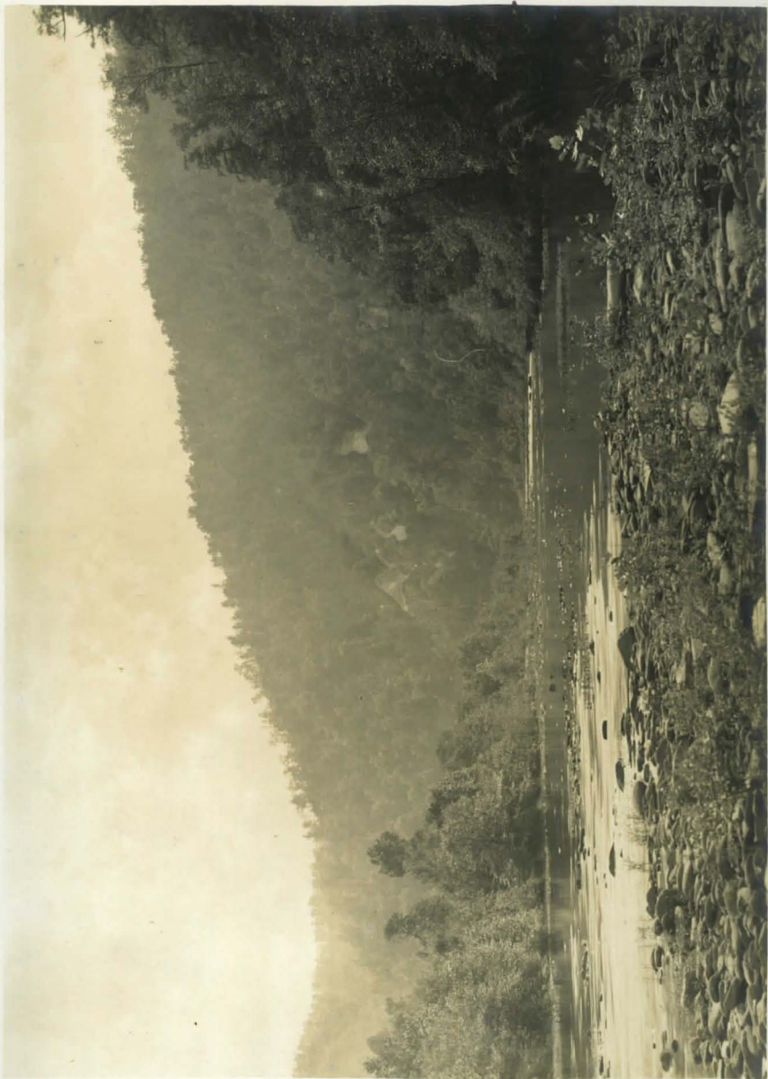
THE HIGHWAY BELOW THE ROUGHS
