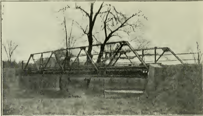
WARREN TRUSS BRIDGE IN MIDDLESEX.
