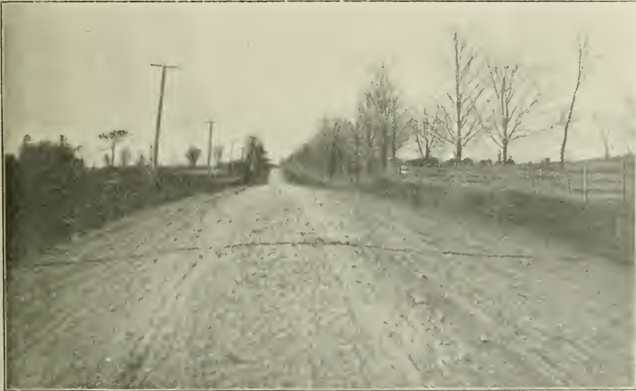
LINCOLN COUNTY STONE ROAD.
