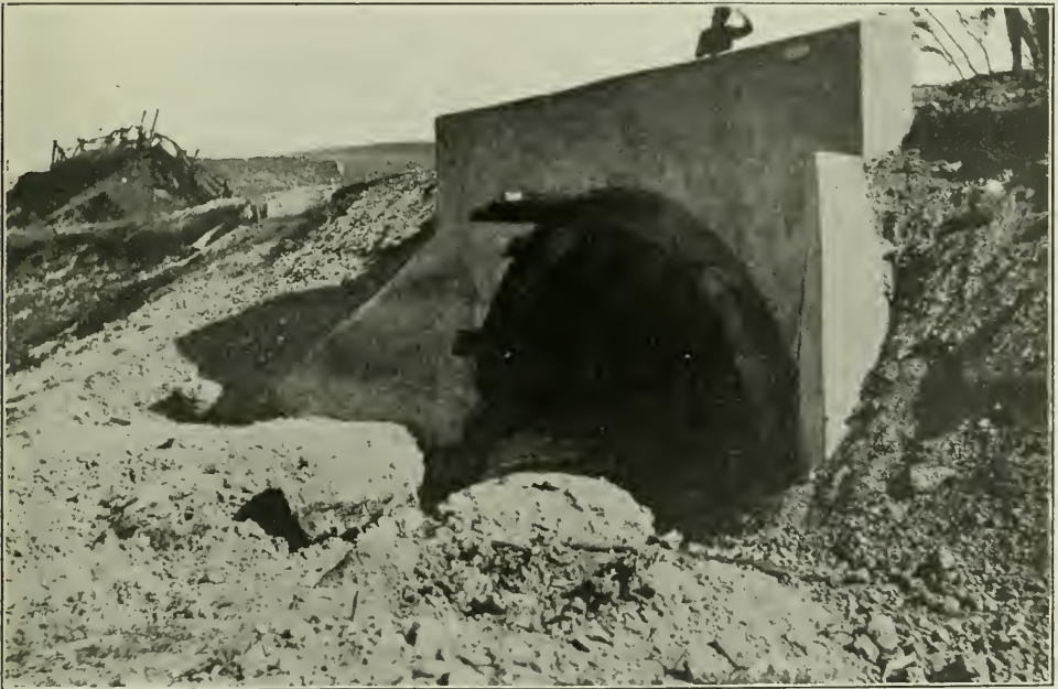
CONCRETE ARCH, SIMCOE COUNTY.
