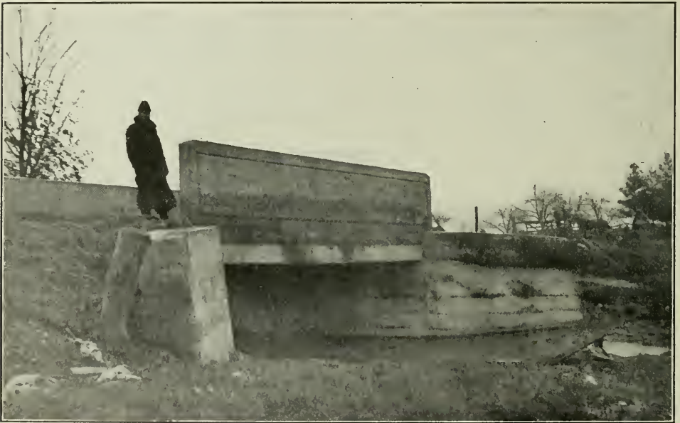
CONCRETE BRIDGE WITH FLAT TOP, MIDDLESEX.
