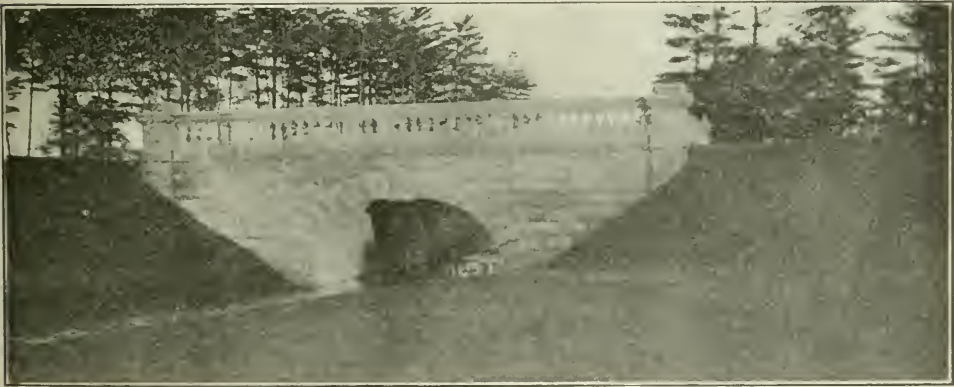
CONCRETE ARCH FACED WITH NATURAL STONE, AT MIMICO.
