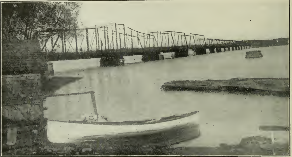
STEEL BRIDGE ON STONE PIERS AND ABUTMENTS.
