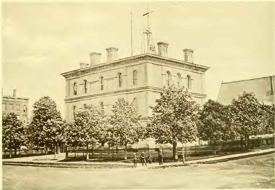
POST OFFICE AND CUSTOM HOUSE.
