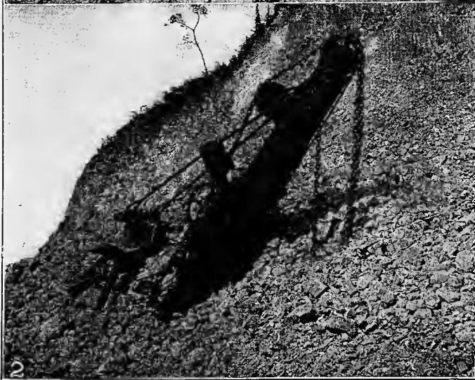
1. STEAM SHOVEL AT WORK. 2. OVERWHELMED BY A SLIDE
