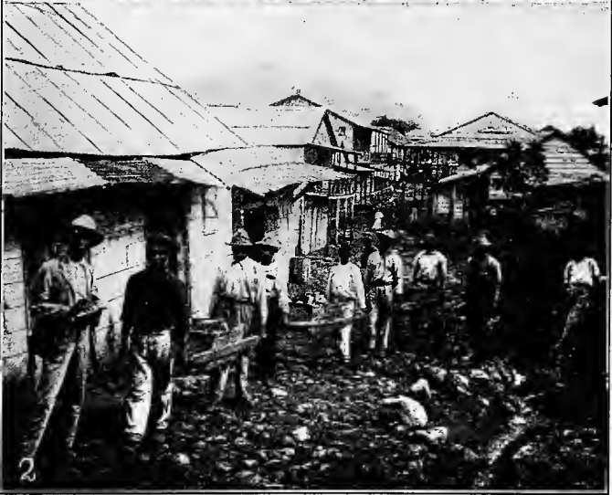
1. AN UNSANITARY ALLEY. 2. BEGINNING SANITATION WORK
