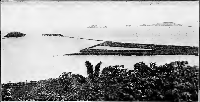
1. ROAD FROM PANAMA TO BALBOA. 2. THE SLICED-OFF ANCON HILL. 3. THE BIG FILL AT BALBOA
