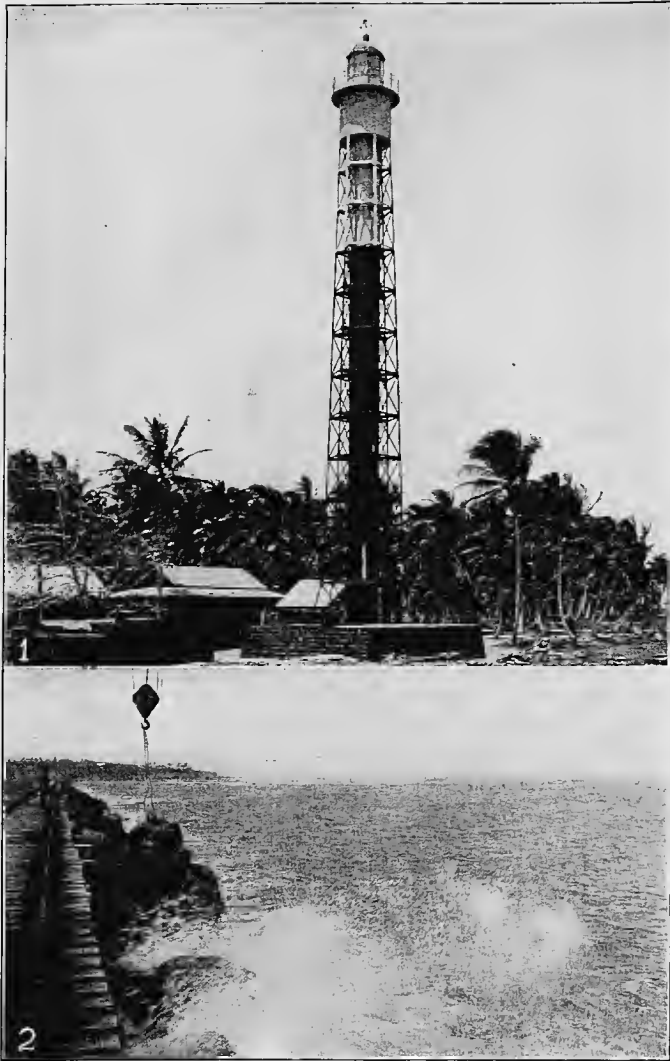
1. TORO POINT LIGHT. 2. TORO POINT BREAKWATER
