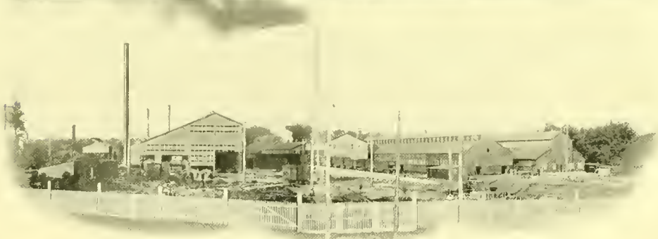
ATLANTA STEEL WORKS END VIEW
