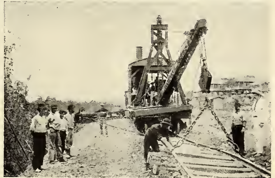
TRACK-SHIFTING MACHINE WHICH LIFTS TIES AND TRACKS TOGETHER.
