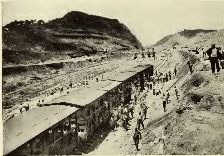
A WORK-TRAIN BRINGING LABORERS TO THE CULEBRA CUT.
