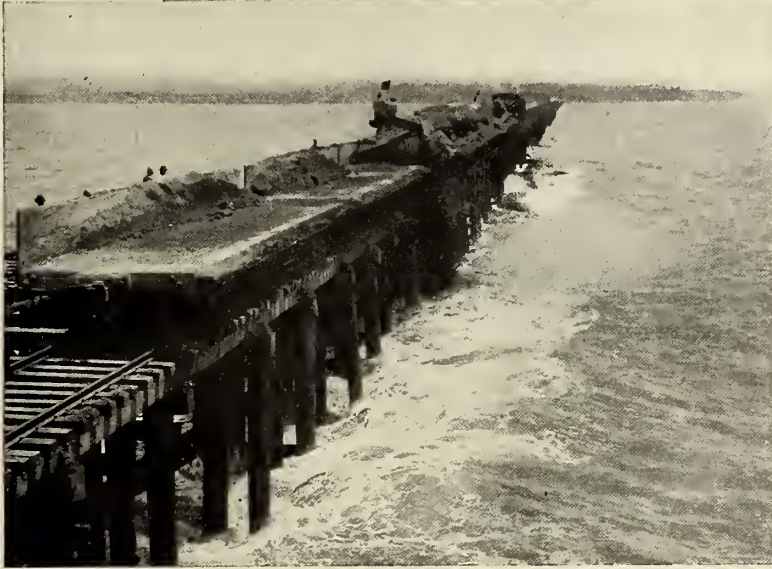
UNLOADING ROCK ON THE TORRO POINT BREAKWATER, AT THE PACIFIC END OF THE CANAL.
