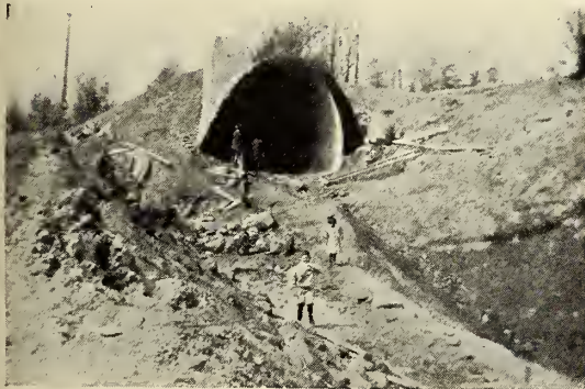
NO. 2. THE AQUEDUCT PIPE.
