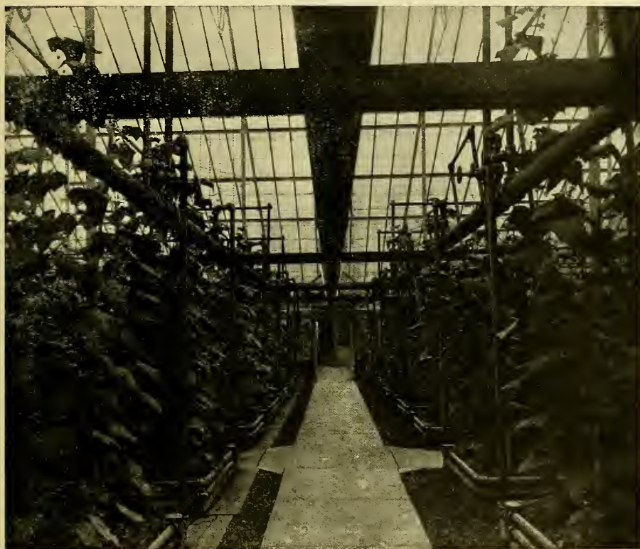
Fig. 20-7. Crosswise view at the center of one of the cucumber houses of the Davis Gardens, showing arrangement of heating coils around the beds
