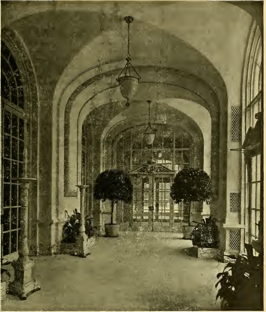
Fig. 10-2. The entry of a modern apartment building showing heat outlets in the side walls.
