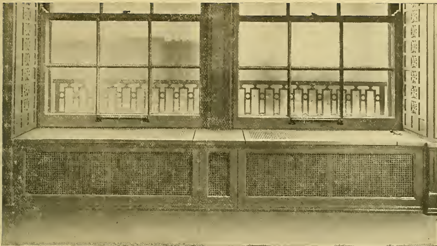
Fig. 6-15. An enclosed radiator in a window seat, with grilles of rattan cane. The Modulation Supply Valve control is placed on the window seat.
