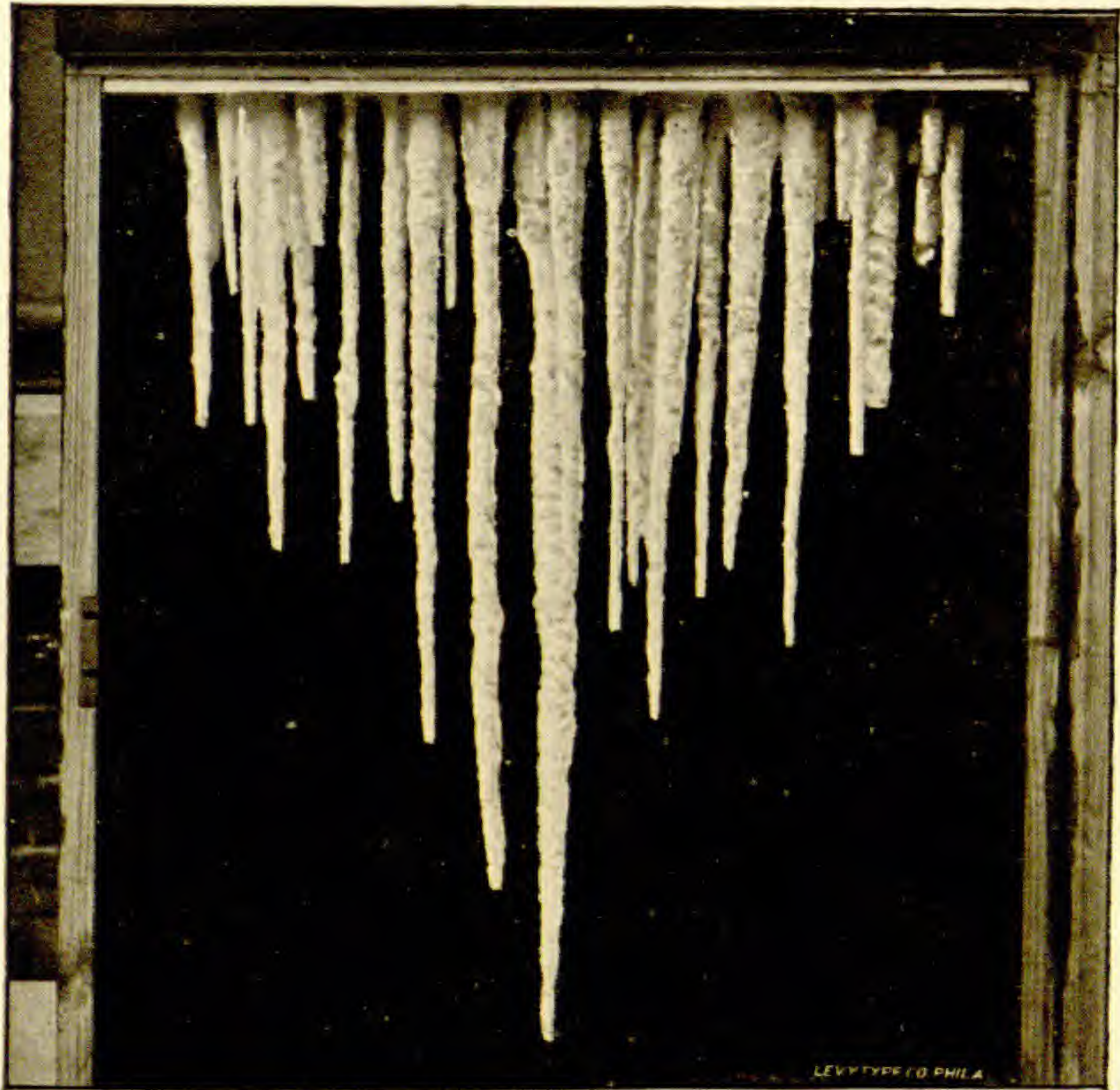
From photograph of Stalactite 60 centimeters long and 20 years old ; formed between the years 1873 and 1893 on the ceiling of a reservoir roof arch at Bayreuth, Bavaria. Scale \frac{1}{7.73}
