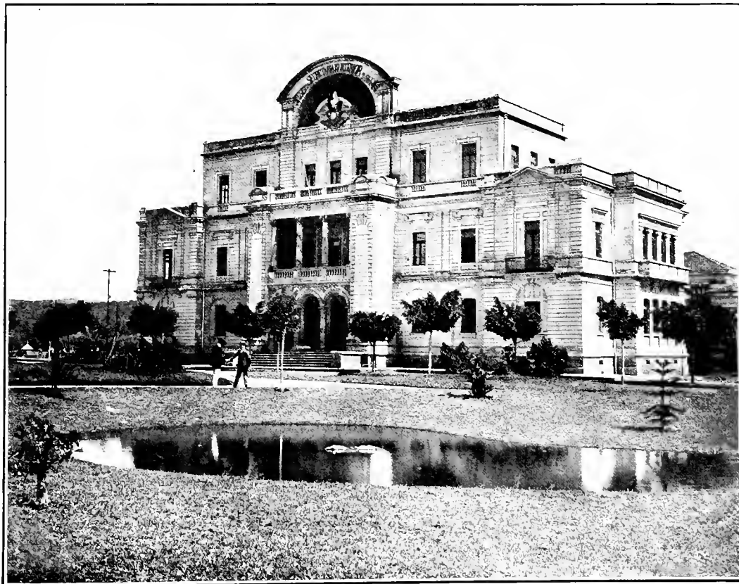
PALACE OF THE DEPARTMENT OF INTERIOR, STATE OF MINAS GERAES.
