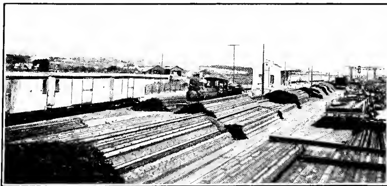
SOROCABANA STATION OF BARRA FUNDA, SHOWING MATERIAL FOR CONSTRUCTION OF THE LINE TO MATTO GROSSO.
