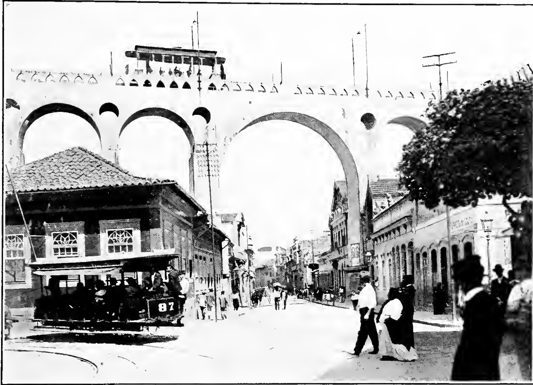
OLD CARIOCA AQUEDUCT SEEN FROM BELOW
