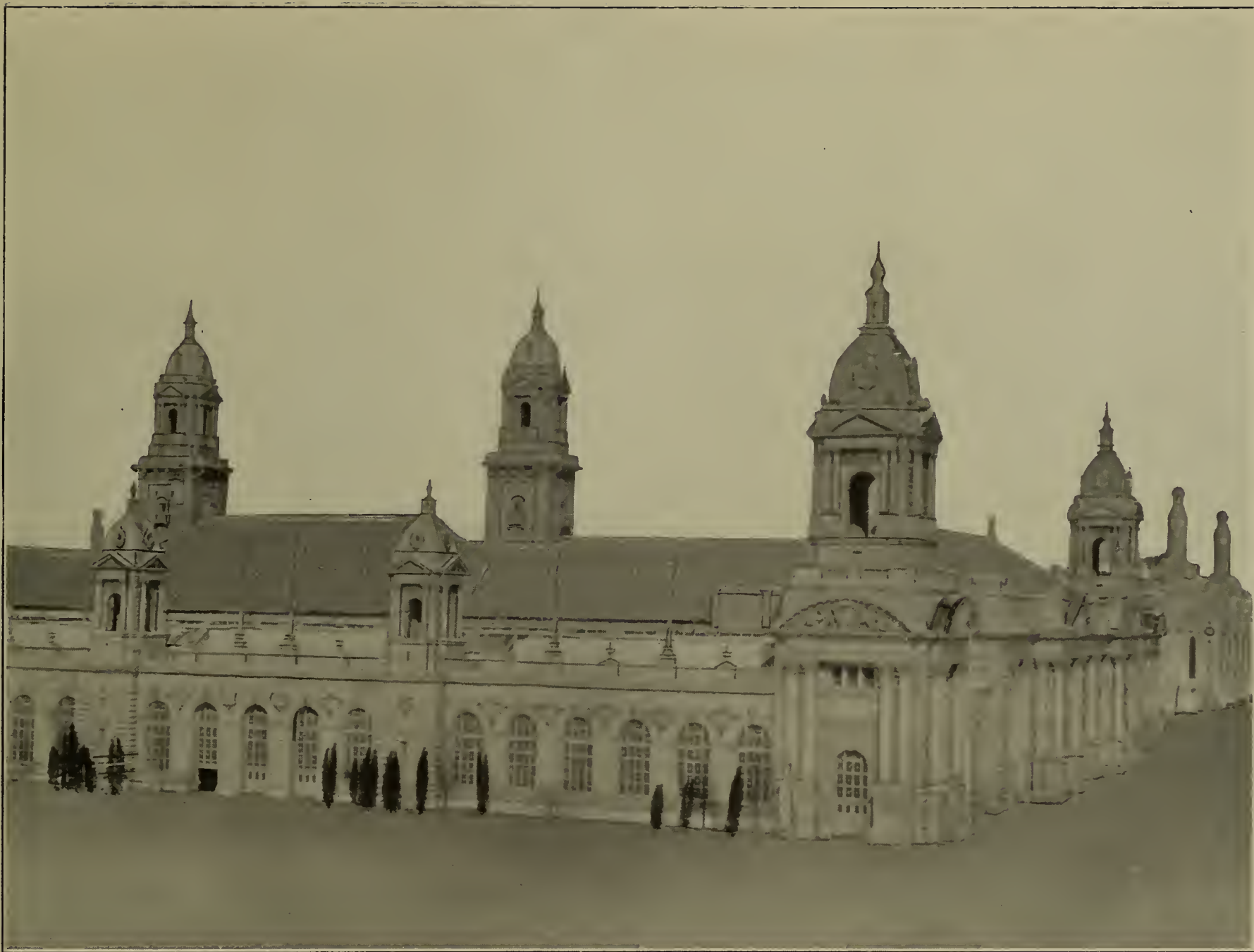
PALACE OF MACHINERY. Size, 525 by 1,000 feet, and cost $500,000. The towers, of which there are seven, are the highest on the Exposition grounds, the two located at the main entrance being 285 feet high. All will be illuminated at night with many thousand electric bulbs, and powerful searchlights will play nightly from the top of each tower. The exhibits will include all manner of machinery and tools; steam, gas, petroleum, alcohol, heated air, and water pressure engines, windmills and wind motors, fire engines, and apparatus.
