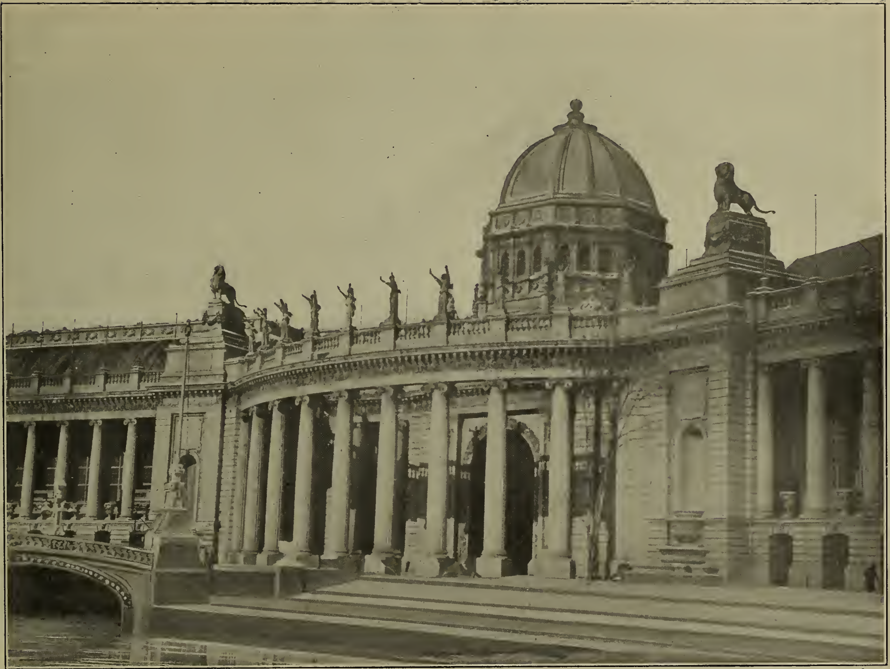
PALACE OF VARIED INDUSTRIES—SOUTHERN ENTRANCE. The beauty of this entrance is unsurpassed in the Exposition. This photograph is a particularly fine one of it, catching, as it has, the light and shade effects, and, taken at just the proper distance, shows the dome which crowns the building.
