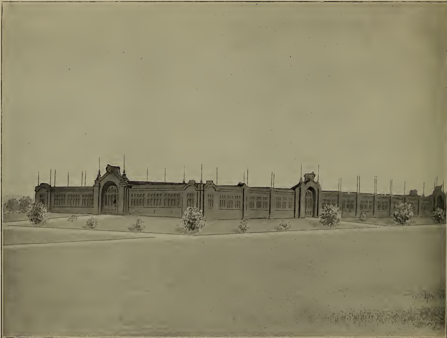
PALACE OF AGRICULTURE. The largest building on the grounds; lies just east of the Philippines, on what is known as Skinker road. Its size is 500 by 1,600 feet, covering twenty acres of ground; cost, $600,000. Agricultural implements and farm machinery, dairies and their fittings, flour mills and methods employed in the preparation of food will be exhibited; also seeds, eggs, cheese, butter, vegetables, fruits, wines, as well as cereals of all descriptions.
