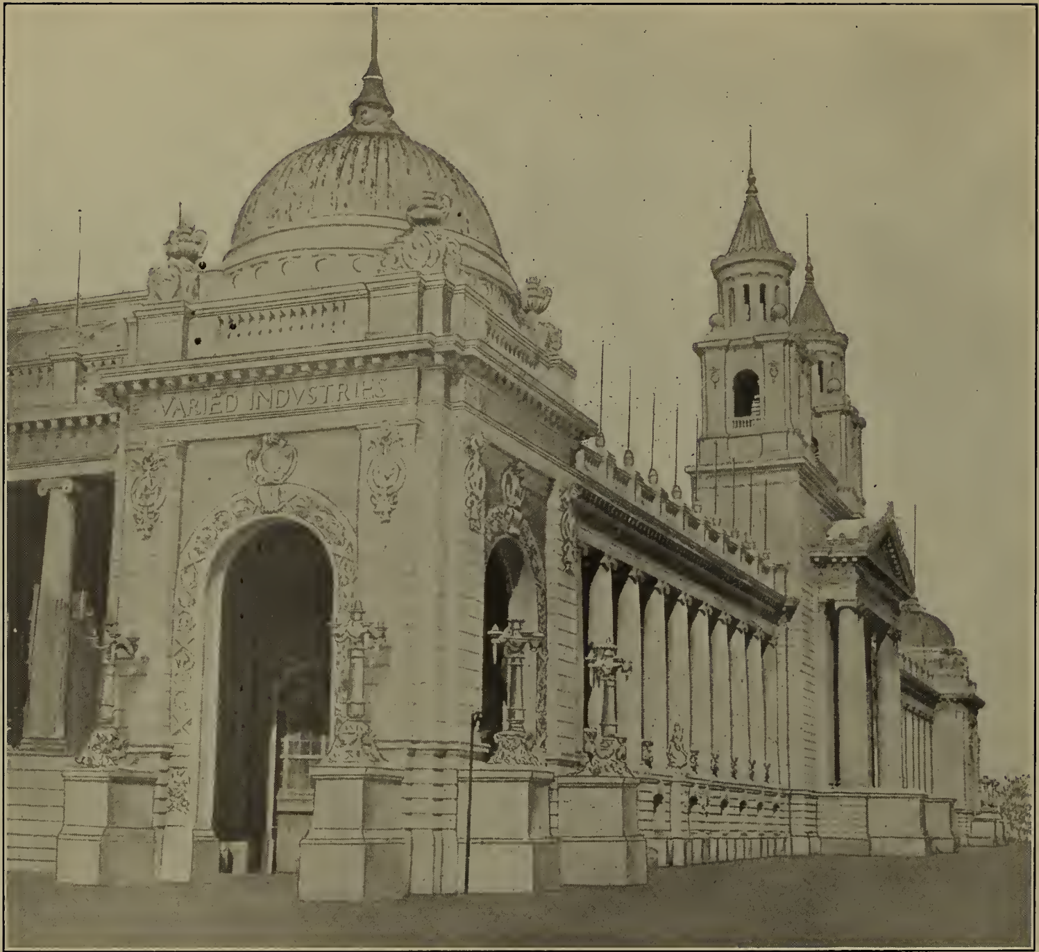
PALACE OF VARIED INDUSTRIES—EAST SIDE.
