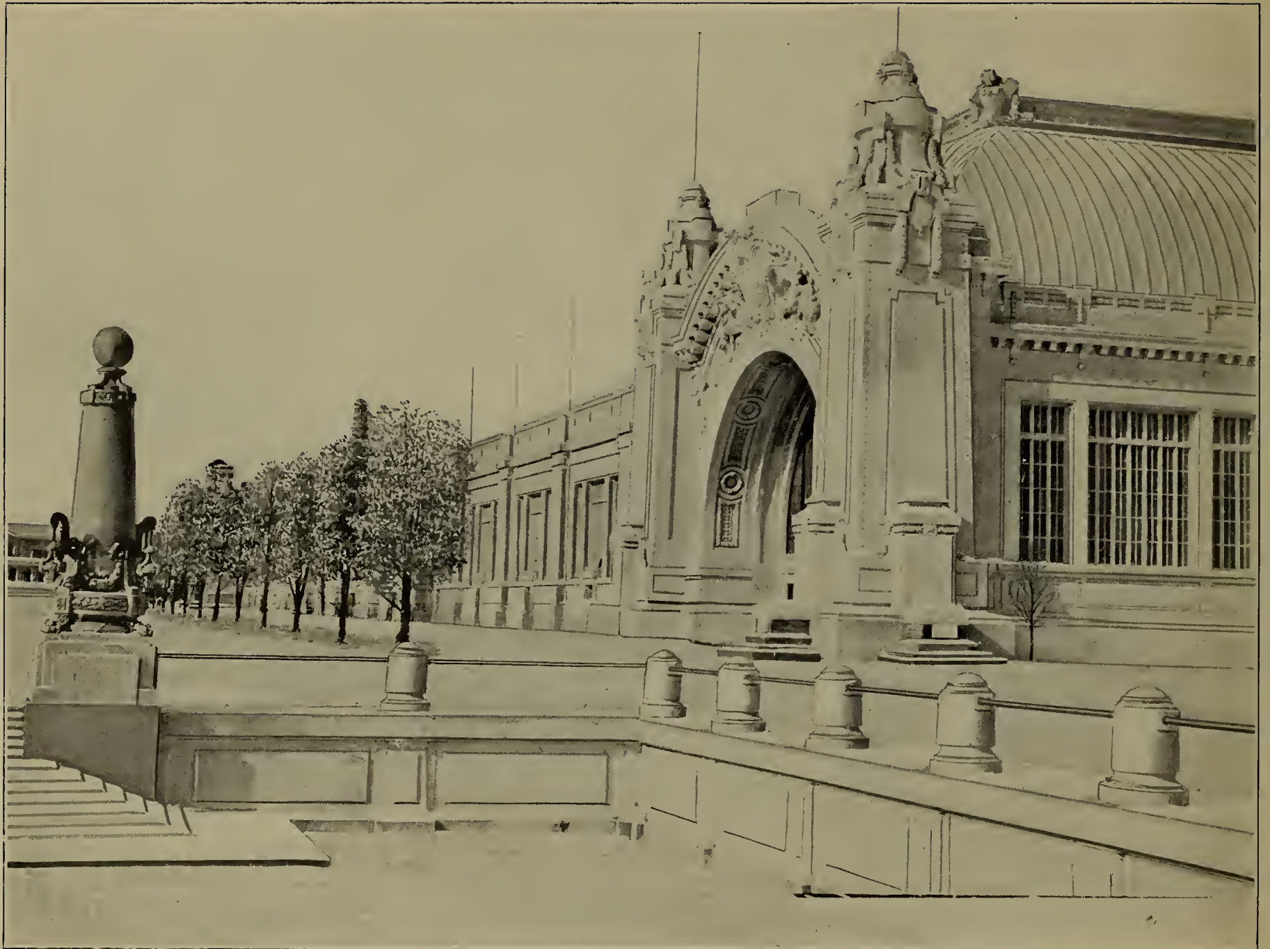
PALACE OF TRANSPORTATION—SOUTH FRONT.
