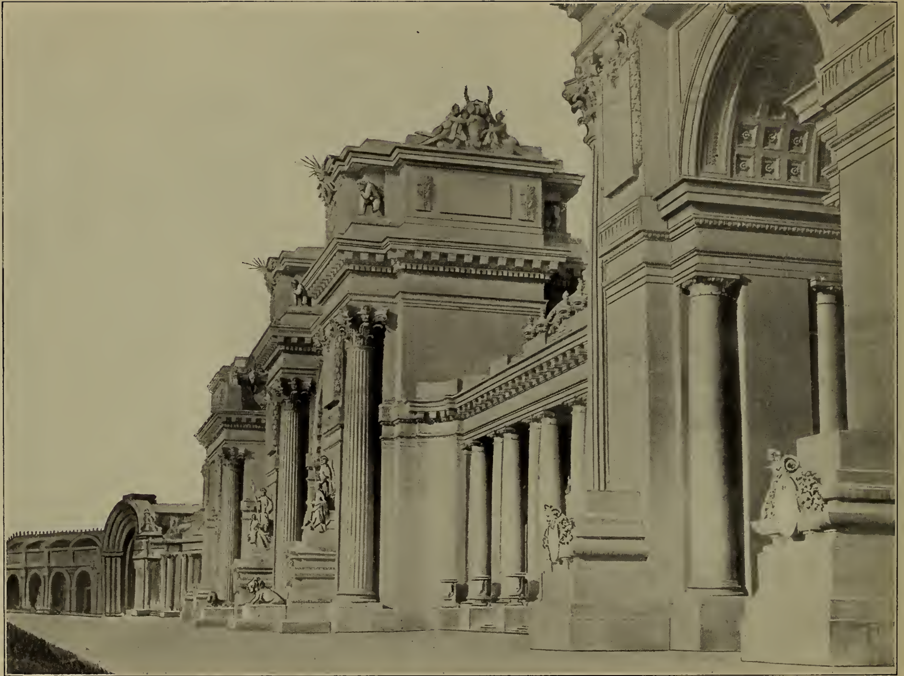
PALACE OF LIBERAL ARTS—WEST FRONT. The main facade is 750 feet long and 525 feet wide; cost, $475,000. The machinery and equipment used in various printing processes, photography, and book making will be here exhibited; also the manufacture of coins and metals, mathematical and scientific instruments, musical instruments, and those used in civil, military and architectural engineering. A novel exhibit will be the printing of an eight-page newspaper daily, giving the news of the day, particularly the happenings at the Exposition, on one of the latest newspaper printing presses, where 240 eight-page papers will be turned out each minute.
