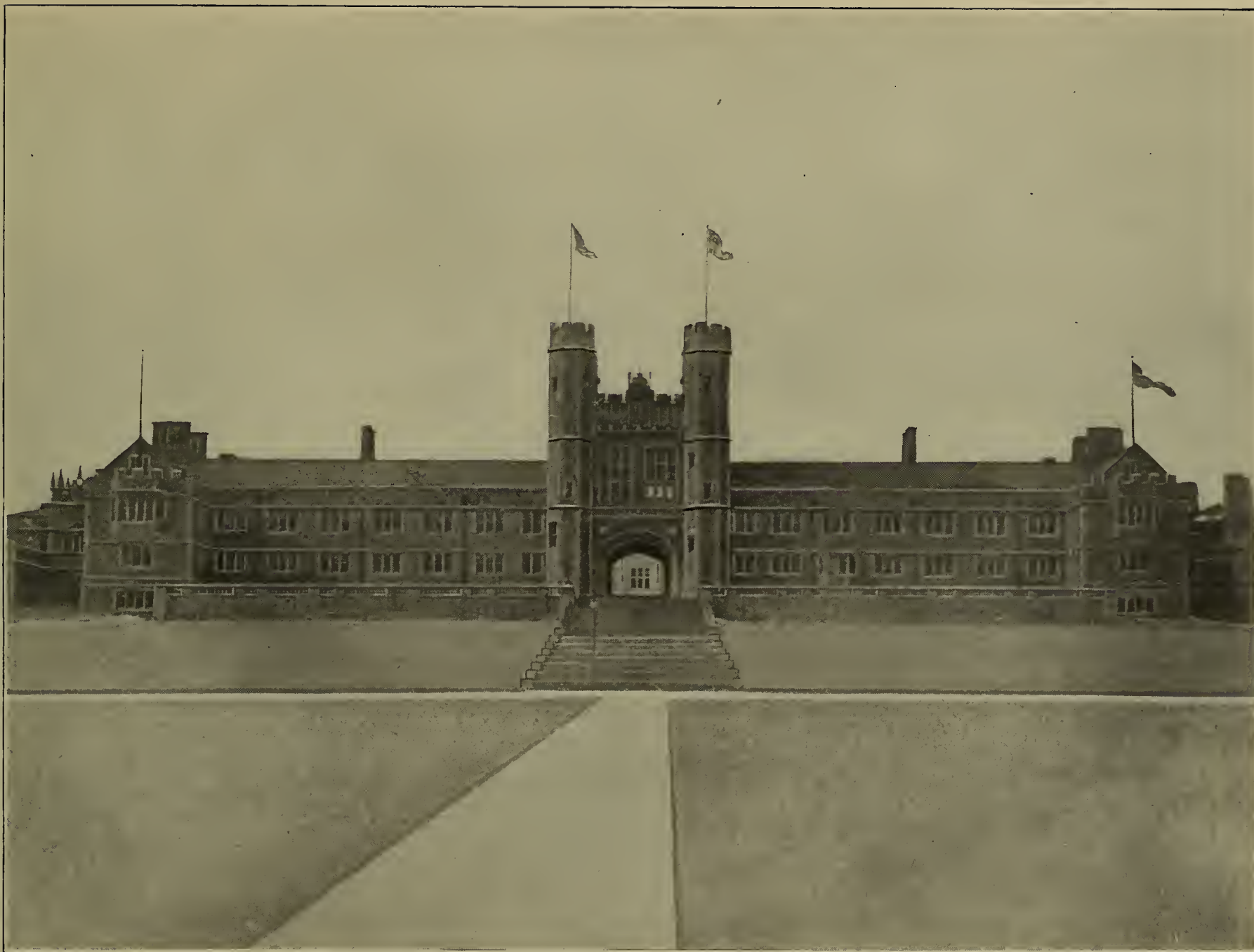
ADMINISTRATION BUILDINGS. These buildings, or rather group of buildings, are built of red granite, with limestone ornamentation, and cost about $1,500,000. They are used exclusively by the officers and the clerical force attached to the administration of affairs of the Exposition. There is a magnificent library in the building.
