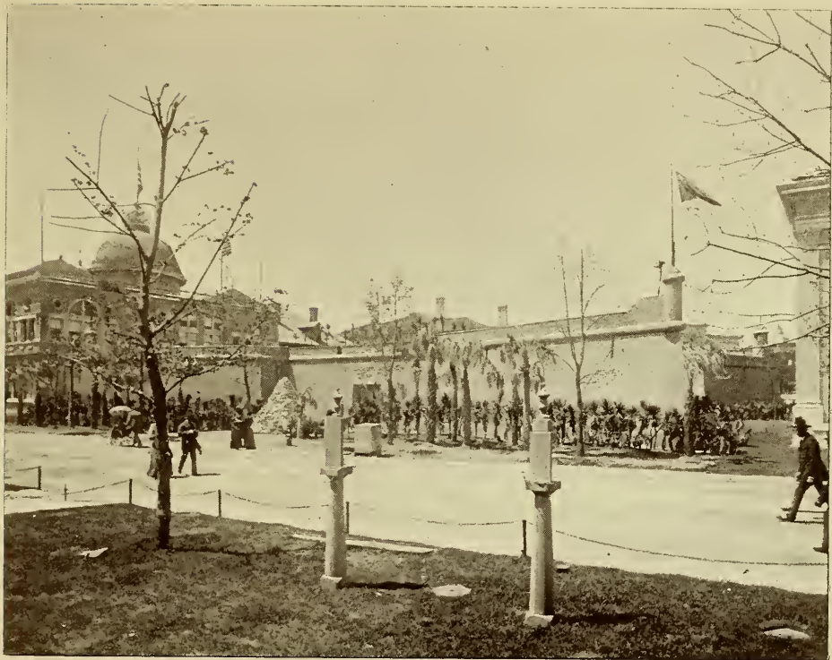
FLORIDA STATE BUILDING.
